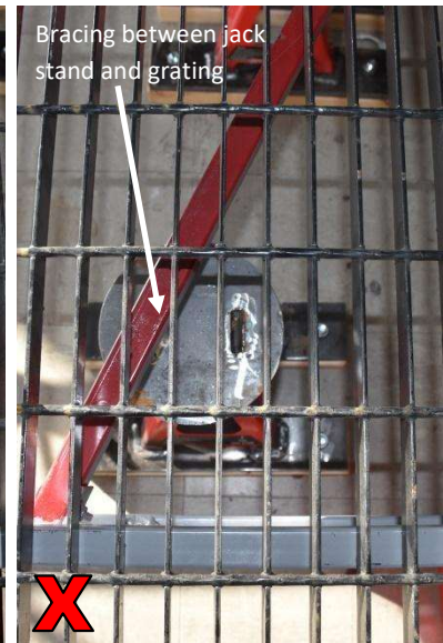
Figure 6b. Incorrect position.
