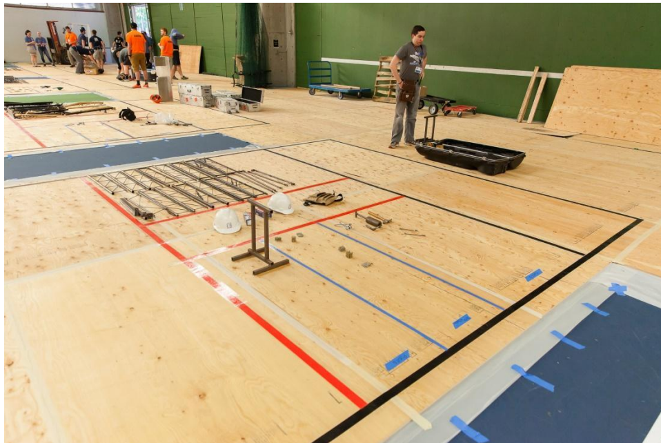
Staging area with bridge ready to go
