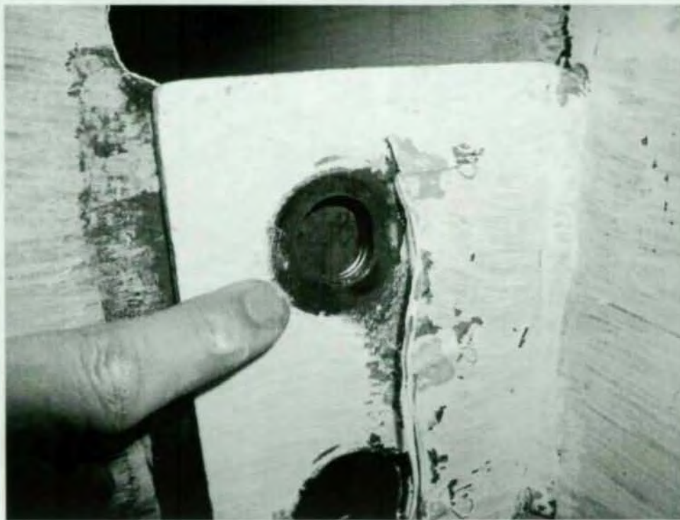
Test 6A – Top Bolt Hole in Shear Tab at End of Test
