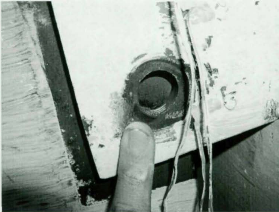
Test 6A – Bottom Bolt Hole in Shear Tab at End of Test
