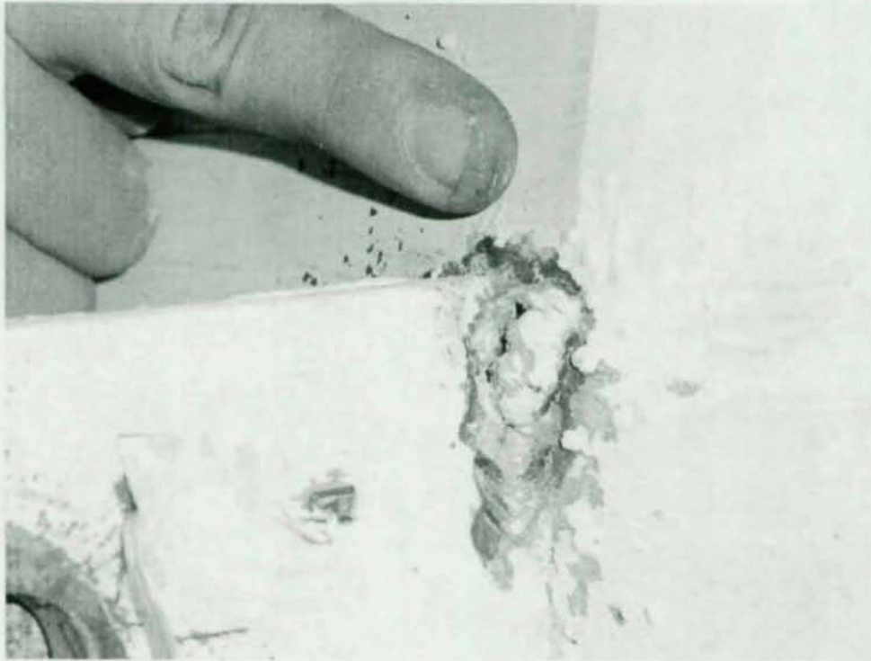
Test 7A – Failure of Shear Tab Weld at End of Test
