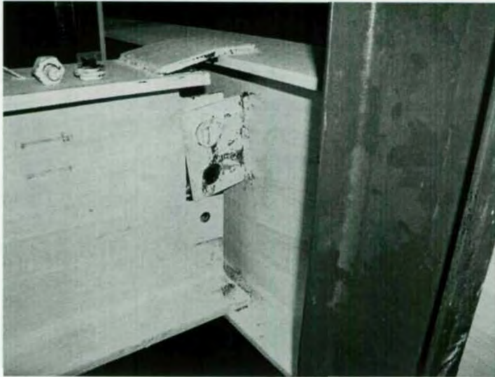
Test 8A – Connection Region at End of Test
