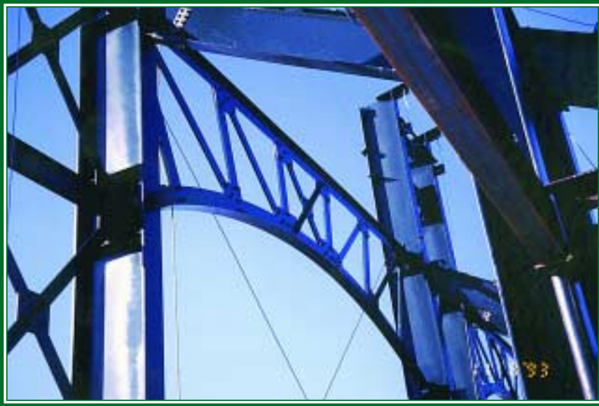
Pictured is the upper concourse grandstand frame during construction.
