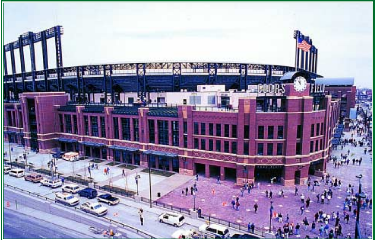
The use of masonry and exposed steel helps the new baseball stadium fit in with the surrounding formerly industrial neighborhood.
