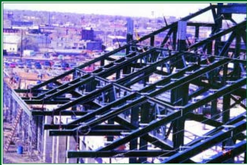
Pictured are the right field mezzanine raker frames.
