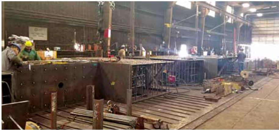
Figure 1. SpeedCore panel module in fabrication. Courtesy of Magnusson Klemencic Associates.
