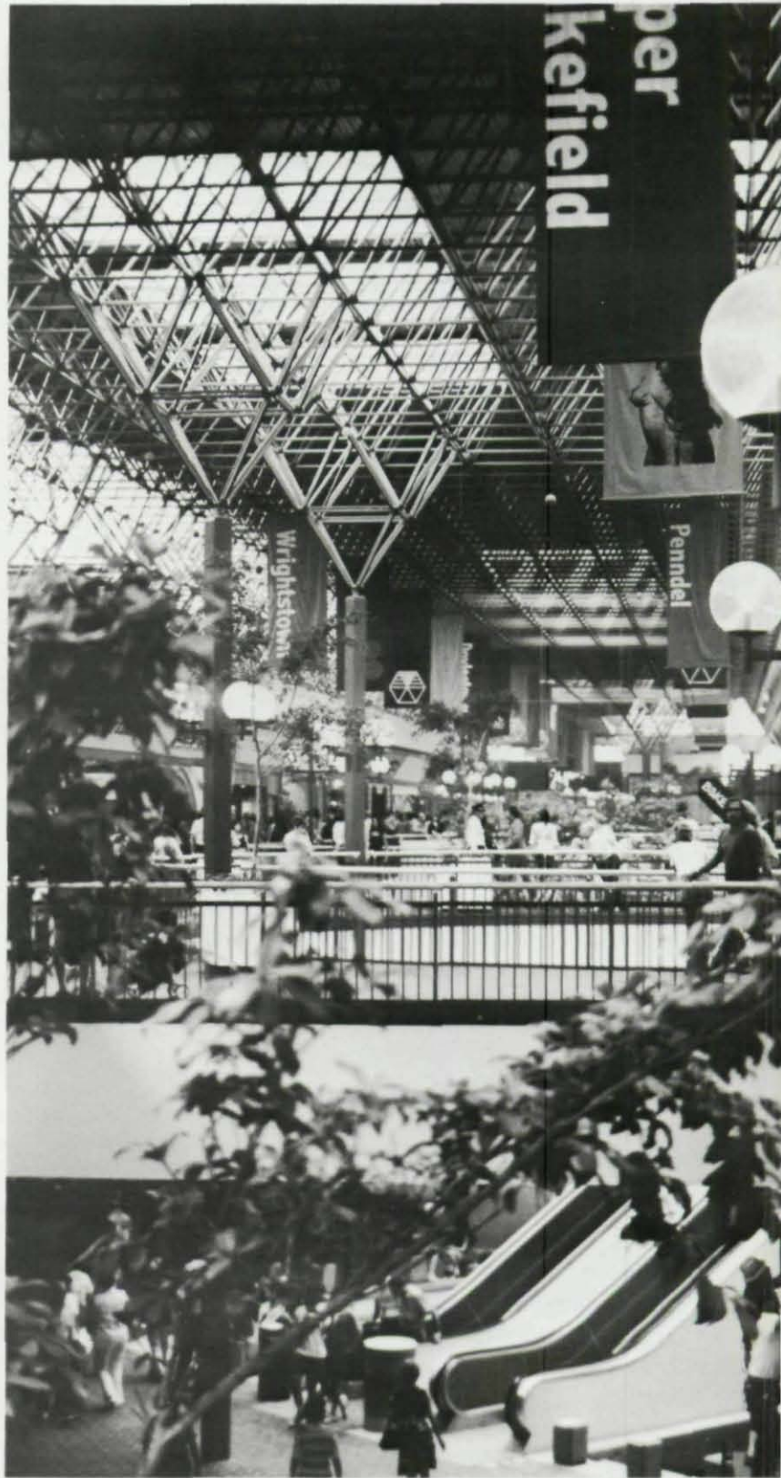
"Here is a fine example of the internal common space which is restoring a very important sense of community to the urban areas of our cities. Steel is a most important material for creating the crystal palace effect that envelops these malls."—Jurors' Comments
