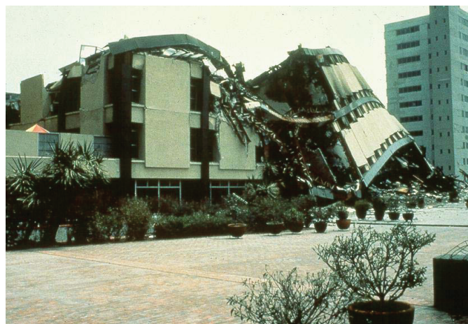
Fig. 2-13. Collapse of the Piño Suarez Towers, 1985 Mexico City earthquake. (Photo courtesy of John Osterass)
