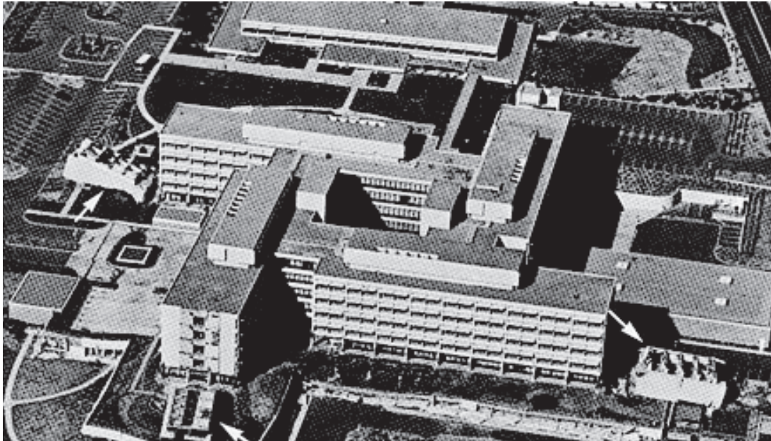
Fig. 10-4. Partial collapse of the Olive View Hospital, 1971 San Fernando earthquake. (Photo courtesy of U.S. Geologic Survey)
