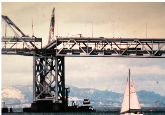
Fig. 2-12. Partial collapse of the Oakland–San Francisco Bay Bridge, 1989 Loma Prieta earthquake. (Photo courtesy of P. Yanev)
