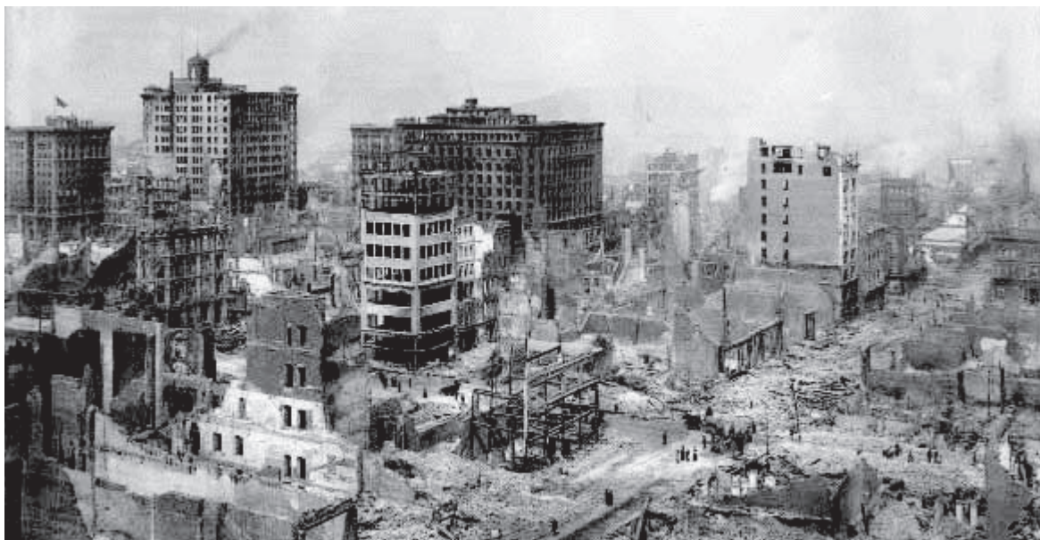
Fig. 10-2. Downtown San Francisco following the earthquake and fires of 1906. (Photo courtesy of Library of Congress)
