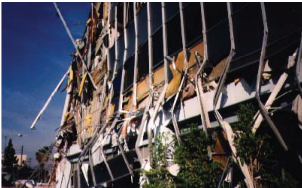
Fig. 2-14. Single-story collapse of the Kaiser Permanente Office Building, 1994 Northridge earthquake. (Photo courtesy of P. Yanev)
