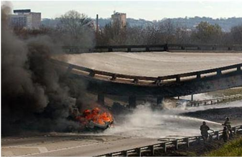
Figure 6 Fuel Truck Crash causes Severe Fire under I-65 South over I-65 North overpass in Birmingham, Alabama, January 2002
