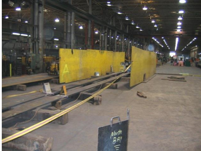
Figure 1 Photo showing the radiographic testing (RT) of a complete joint penetration weld (CJP) with clear area and shielding provided
