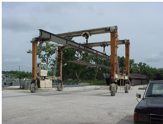
Figure 10 Photo showing overhead gantry type cranes handling material
