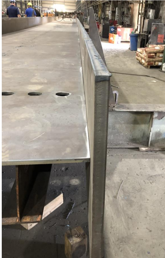
Figure 9 Photo showing the building of girders with its web horizontal
