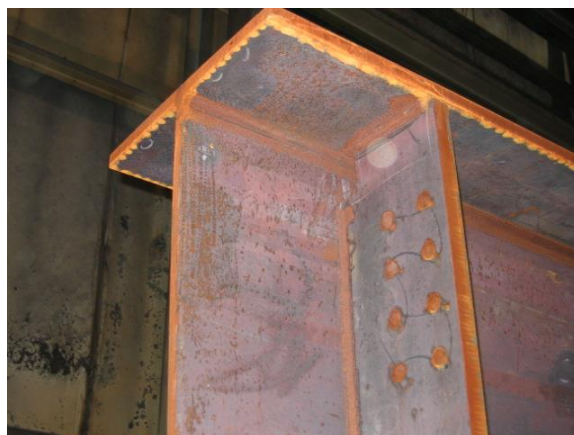
Figure 16 Photo showing a girder before blast cleaning
