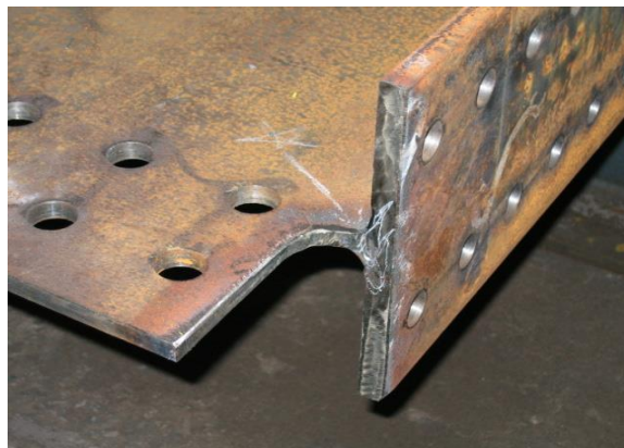
Figure 13 Photo showing an example of a coped girder web and flange
