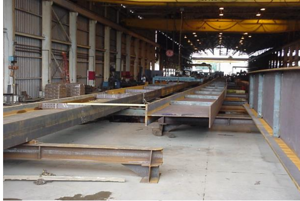
Figure 12 Photo taken in a fabrication shop showing the fitting of transverse stiffeners
