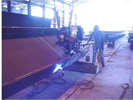
Figure 11 Photo showing the welding of a plate I-girder web to its flange
