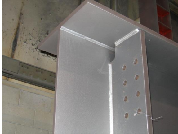
Figure 17 Photo showing a girder after blast cleaning
