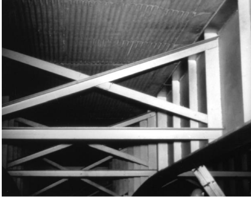
Figure 14 X-Bracing and Girders
