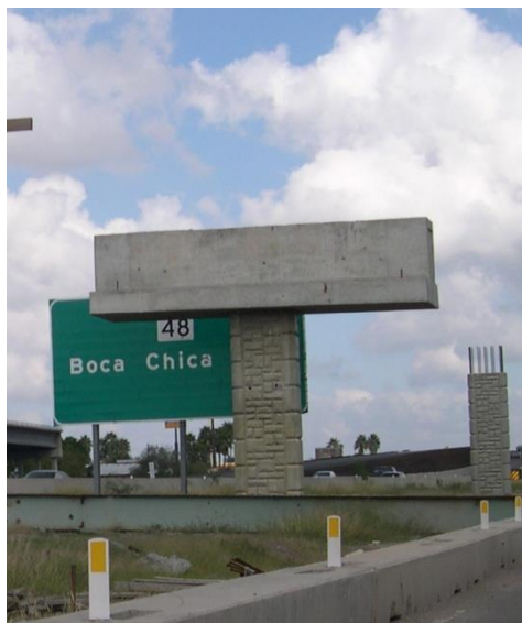
Figure 21 Single column hammerhead pier with an inverted T pier cap.
