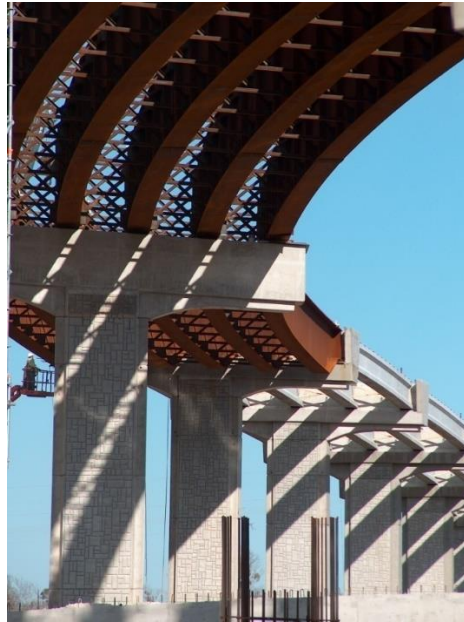
Figure 30 Dapped girder ends rest on an inverted T pier cap in a single column pier.
