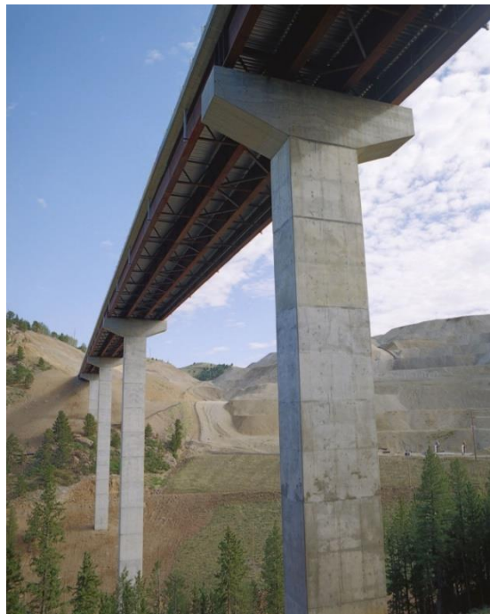
Figure 20 Single column hammerhead pier with tall columns over a deep valley.
