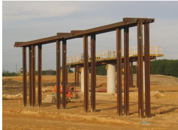
Figure 3 Driven steel H-piles.
