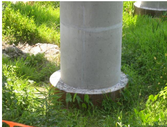
Figure 7 Single round column with an oversized, steel cased, drilled shaft.
