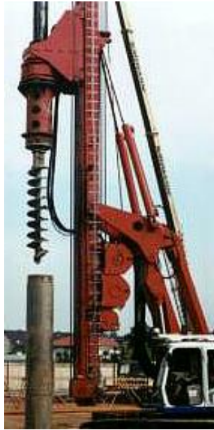
Figure 8 Drilled shaft drilling rig.
