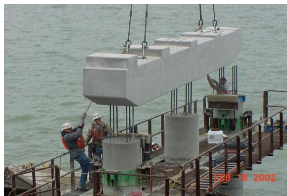
Figure 32 Setting of a precast pier cap.
