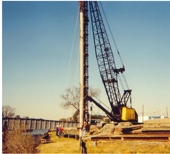
Figure 4 Driving of a precast concrete pile.
