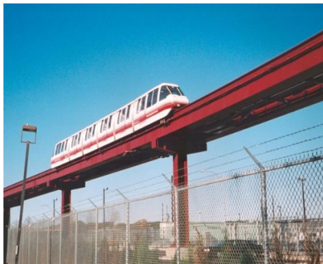
Figure 28 Steel single column hammerhead piers for a dual steel box girder bridge.
