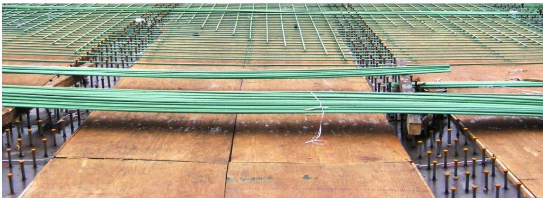
Figure 6 Photo showing temporary wood formwork installed on a steel plate I-girder bridge.
