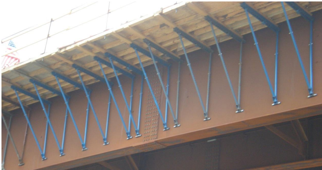
Figure 7 Photo showing deck overhang brackets supporting cantilever slab construction on a steel plate I-girder bridge.
