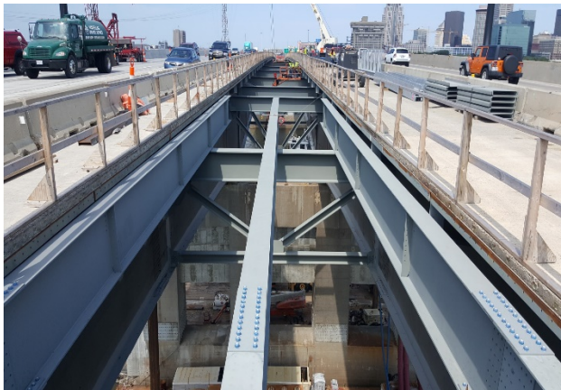
Figure 10: Structural Steel Infill
