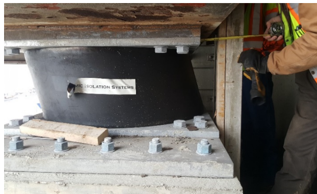
Figure 18: Seismic Isolation Bearing
