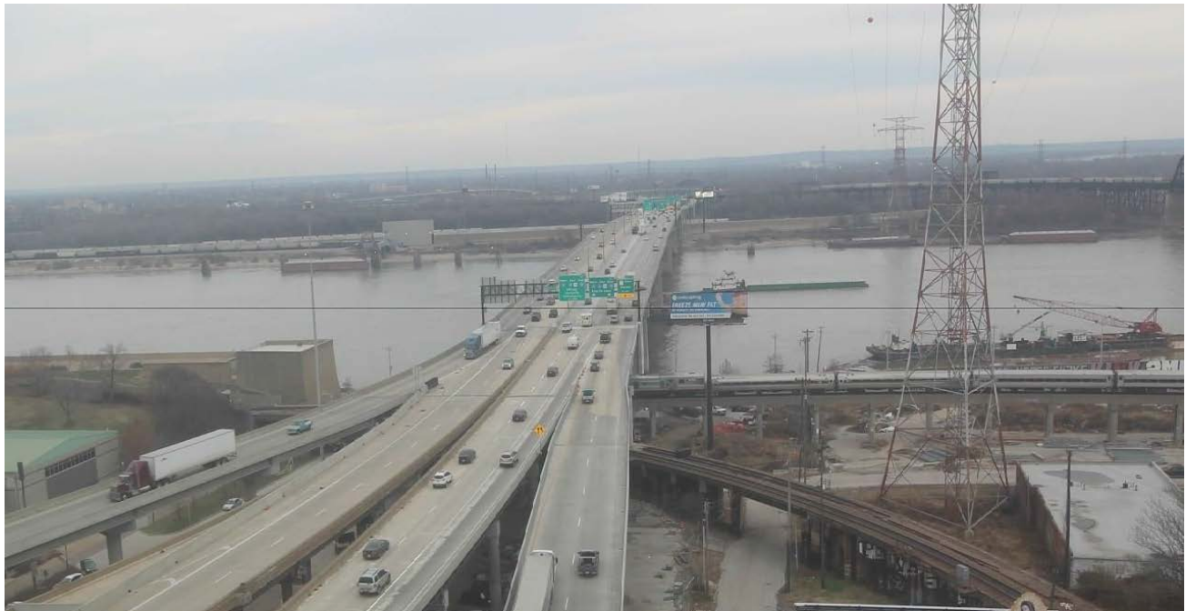
Figure 19: Completed Poplar Street Bridge
