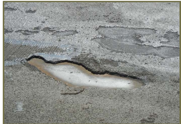
Figure 11: Failed Overlay
