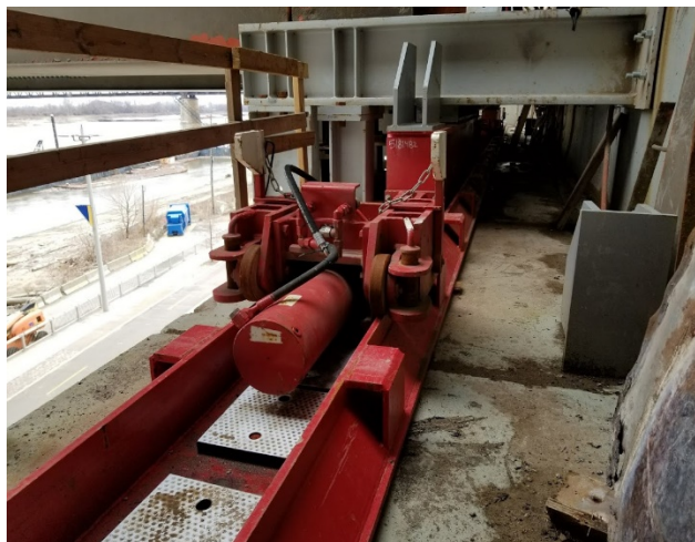
Figure 8: Slide Track System
