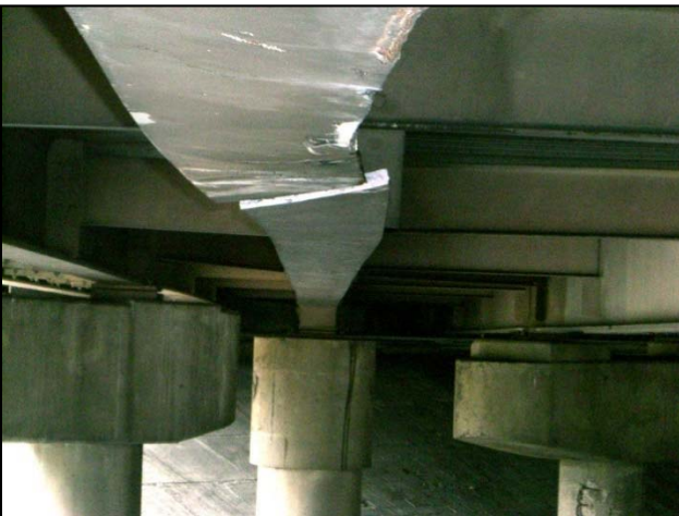
Figure 12: I-66 EB, Span 2 Beam #22, Collision Damage (Split Beam)
