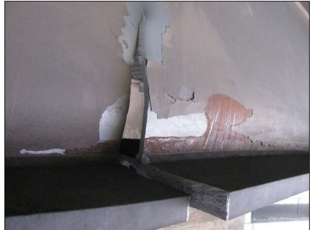
Figure 13: I-66 EB, Span 2 Beam #22, Collision Damage (Split Beam)
