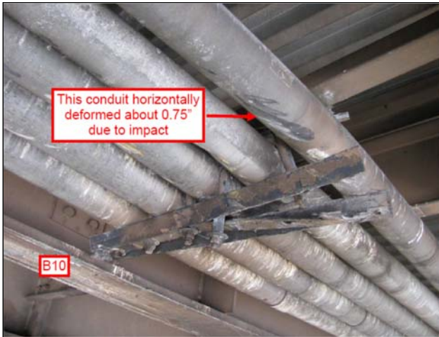
Figure 11: I-66 EB, Span 2, Damaged Utility Hanger
