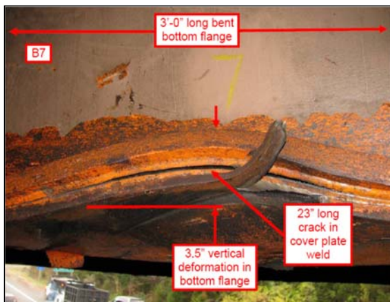
Figure 8: I-66 EB, Span 2 Beam #7, Crack in Cover Plate Weld
