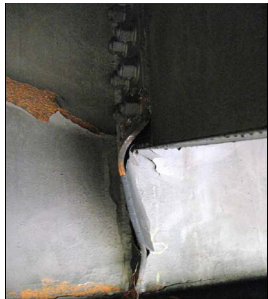
Figure 10: I-66 EB, Span 2 Beam #6, Buckled Connection Plate
