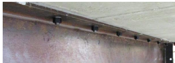
Figure 14 – Installed Adhesive Anchor Connectors
