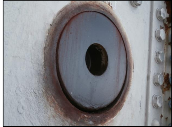
Figure 5 – U29 Lower Pin Downstream Truss Inside Face
