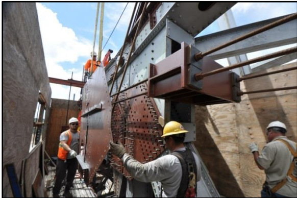
Figure 29 – Splice Plate Template
