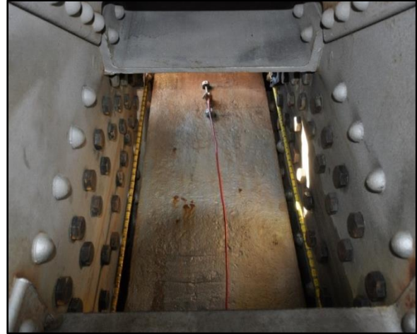
Figure 35 – Wire Saw Inside Truss
