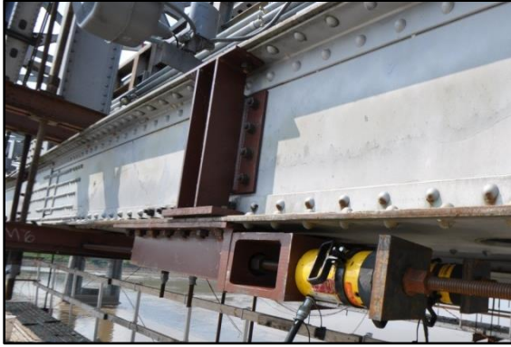
Figure 33 – Lower Longitudinal Restraints
