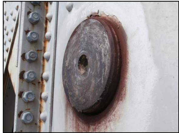
Figure 6 – U29 Lower Pin Downstream Truss Outside Face
