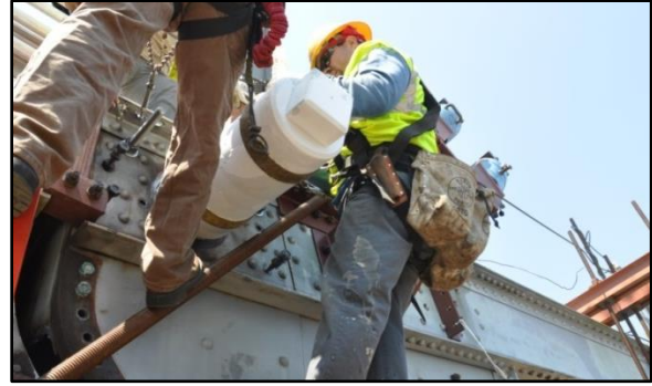
Figure 38 – Installation of New Pins
