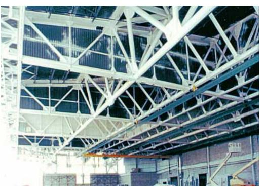
are located through the facility. To enhance flexibility and reduce space, upward acting fabric hangar doors were used requiring special structural details.
