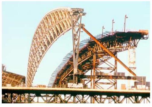
porting position. The trusses also changed position as the secondary framing and roof panels were added. A sophisticated stability check was performed on all the trusses to ensure they would span in both their temporary and final conditions. The check predicted that roof movements would be 18" vertical at center and 9" horizontally at the ends. Actual deflection was within an amazing 3/8" of that predicted!
