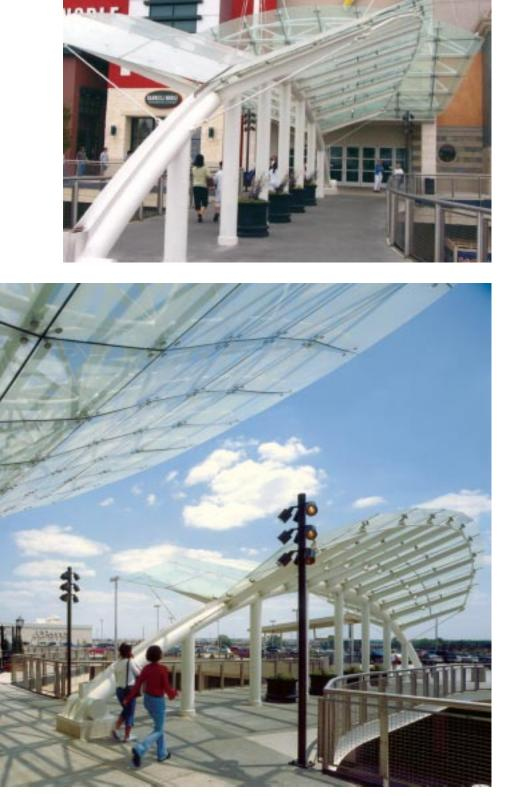
then raised up along its edges. Constructed using a series of king-post trusses assembled from wide-flange steel top chords, HSS compression struts, tension rods, and steel rod bracing, the undulating roof bears lightly on a diagonal HSS truss framing the clerestory glass.
