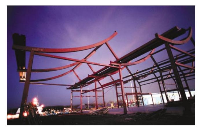
and outside of the project budget. The design team turned to a combination of wide-flange and hollow structural shapes to provide the ideal combination of clean lines, strength and cost effectiveness.
