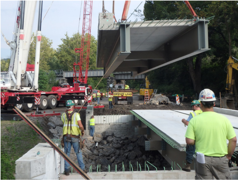
Wampum Bridge, Wampum Borough, Pa. 2016 Prize Bridge Award – Short Span
