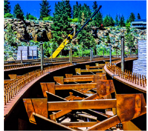
Bill Healy Memorial Bridge, Bend, Ore. Prize Bridge Award – Medium Span
