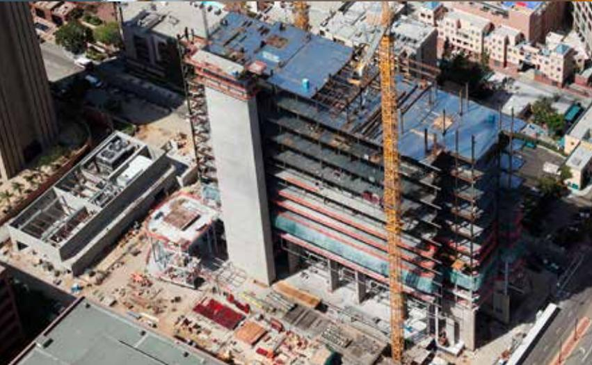
as well as become an ongoing maintenance problem. Using a detailed project schedule developed by the CM-at-risk, the structural engineer developed multi-stage structural models to investigate and discount differential settlement concerns, thereby eliminating the need for a plaza-level joint. (For more on this project, see the June 2013 issue).
