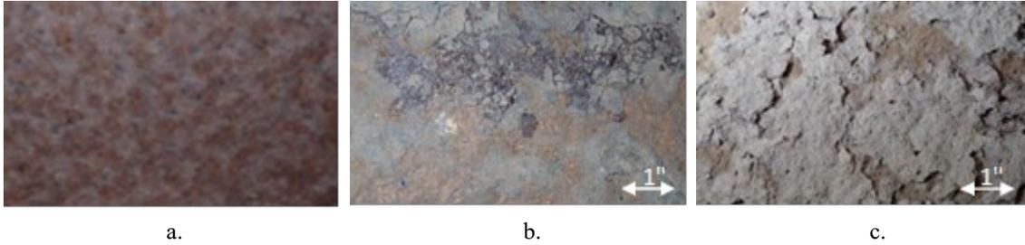
**Figure 4.1.1.2-3—Photographs of poor performance of UWS showing various textures: (a) rough "freckled" surface, (b) a relatively smooth surface that was easily crushed by tapping, (c) coarse surface with exfoliating rust layers.**
