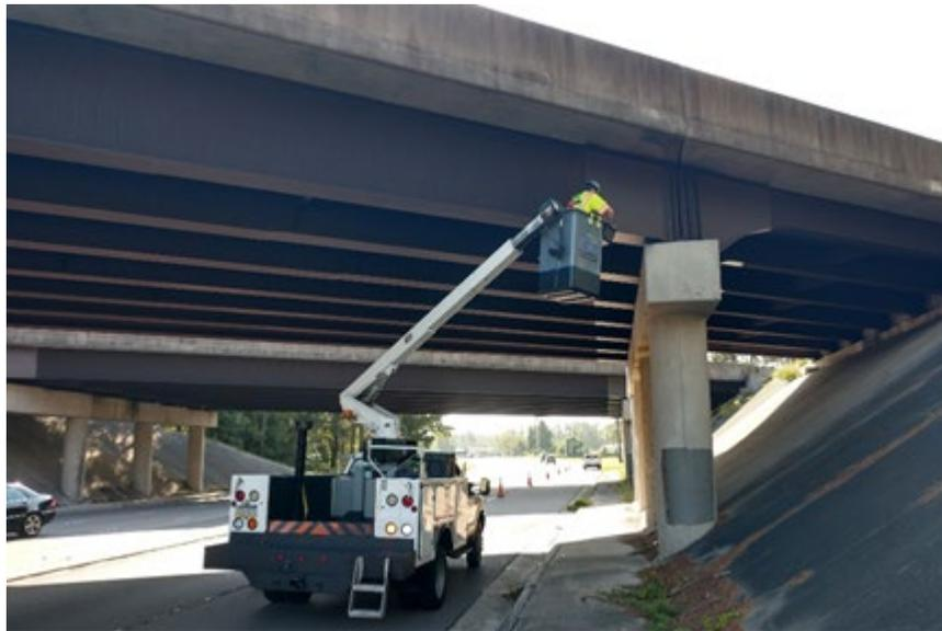
**Figure 1.1.1-1—This 30-year-old bridge two miles from the Atlantic coast is one of thousands of examples of UWS bridges performing well after decades of service.**
