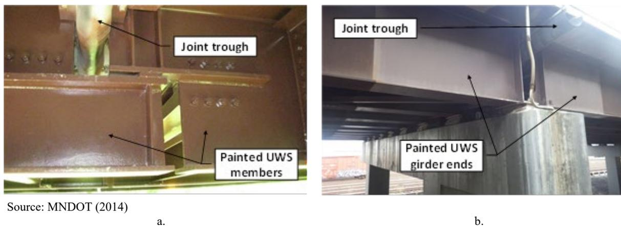
Figure 6.1.1-1—Example painting of UWS members beneath deck joints.
