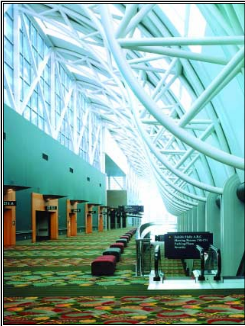
The main concourse features "banana" trusses on one side and "snowflake" X-bracing on the other.
