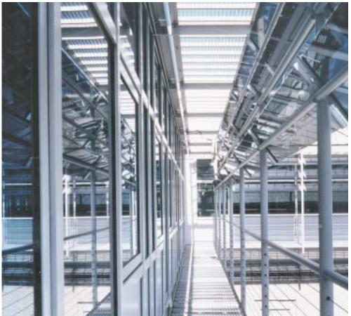
hipped-roof configurations, the roof form not only maximizes solar orientation but creates a breakdown in scale sympathetic with the roofscape of the campus. Each of the 4.8m bays is enclosed by a high-performance curtain wall system and solar control system. The rhythms and color reflect both internal structure and program needs as well as the rhythms of the historic terra cotta facade.
