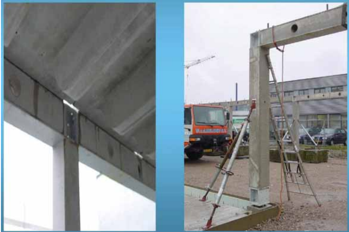
Figure 1: Delftech office building in Delft, the Netherlands; built in 3 weeks time (source: [2])
