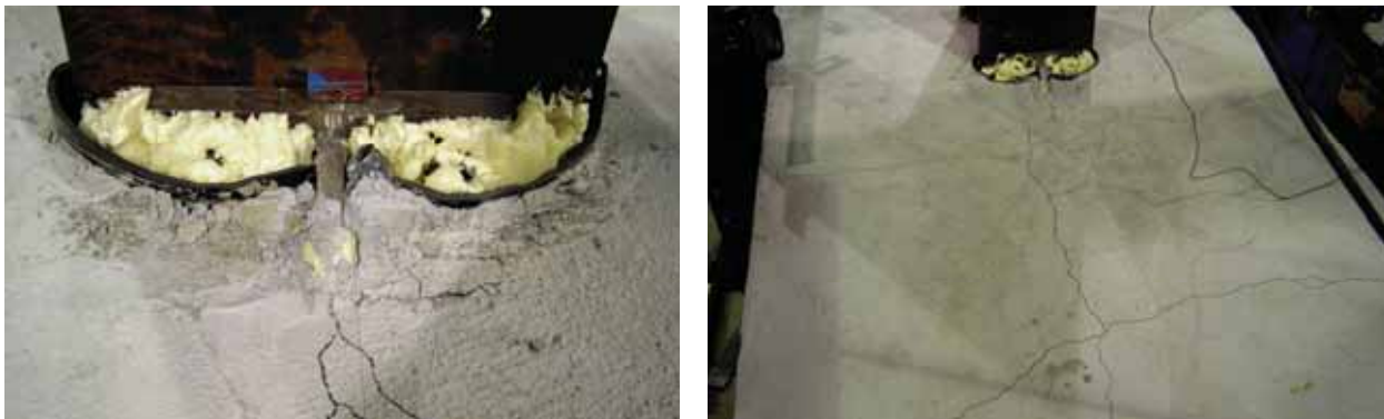
Figure 7. Cracking of Slab
