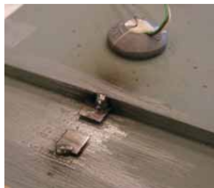
Fig. 5. Ethyl silicate zinc coating appearance
