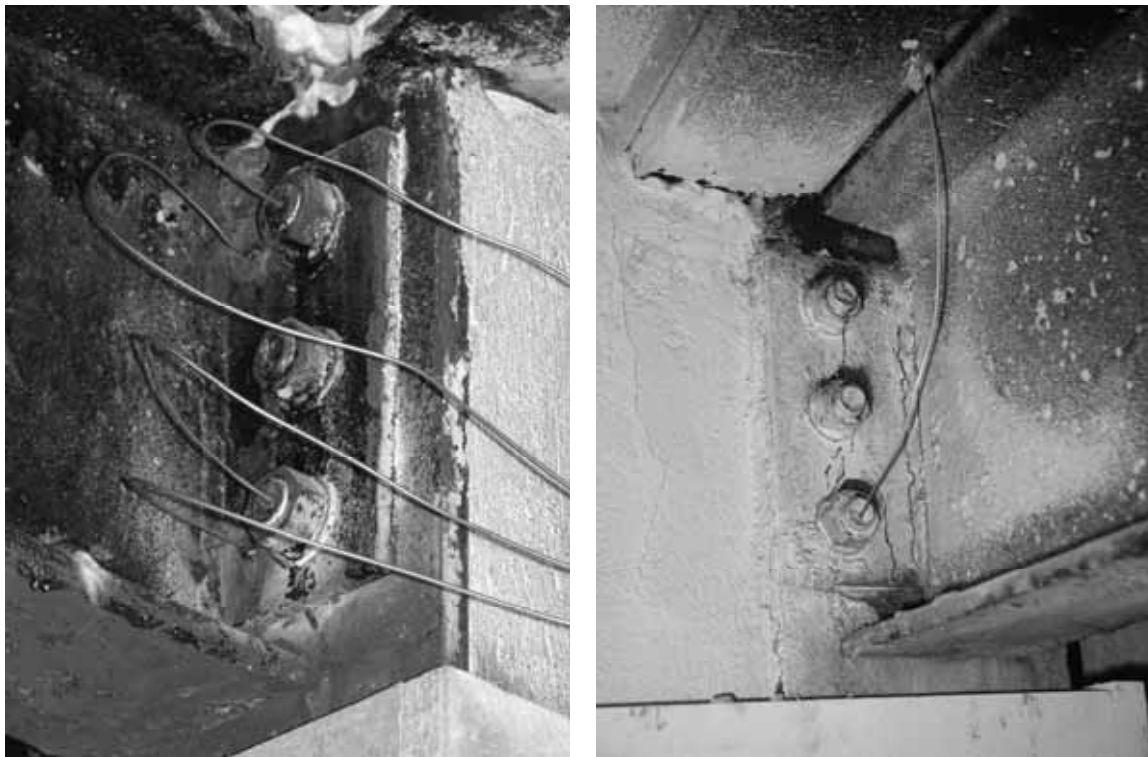
Fig. 2 - Position of the thermocouples on the header plate connections.
