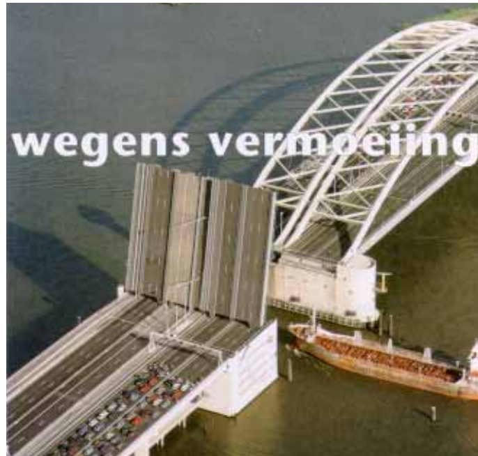
Figure 1. The Van Brienenoord bridges in the main North-South highway in Rotterdam. The words wegens vermoeiing mean because of fatigue .
