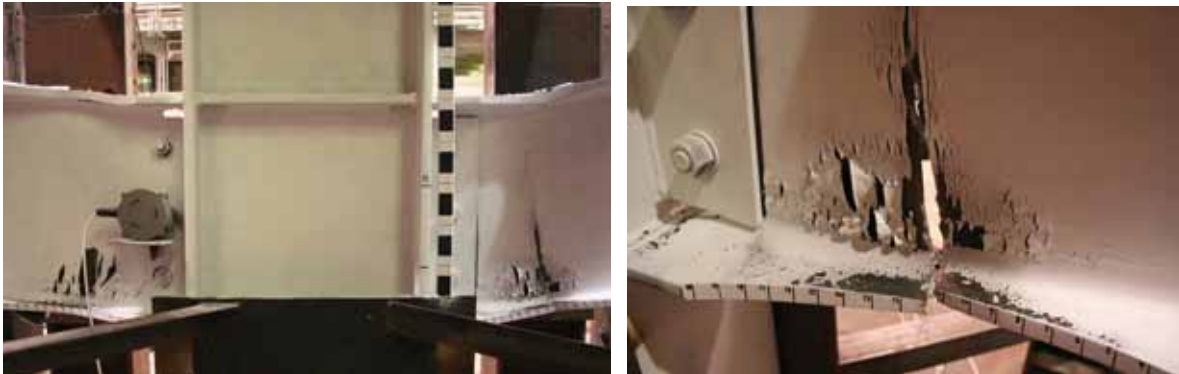
Figure 9: Failure mode of the RBS Test Specimen
