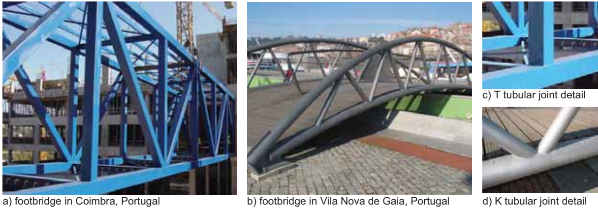
Figure 1. Examples of tubular structures with T and K tubular joints
