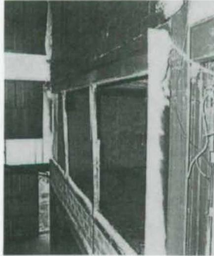
Figure 14 *Windposts following fire*
