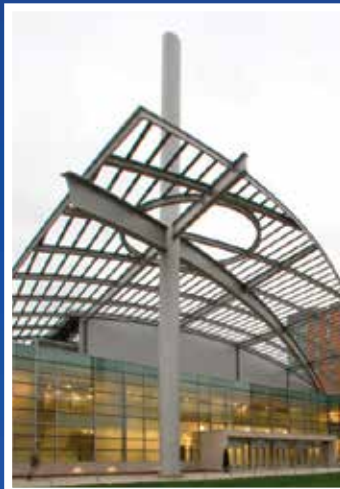
2010 NCSEA Award Winner - 200 tons of beams, channels and angle for the roof of the University of Illinois at Chicago Forum. Chicago, IL
