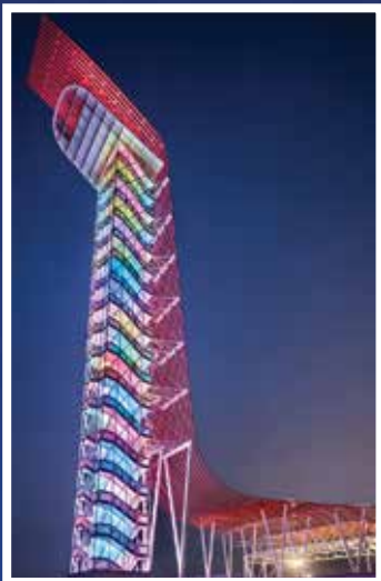
2015 IDEAS 2 Merit Award - 385 tons of 70 curved 8 inch sch 40 pipe for Circuit of the Americas Observation Tower. Austin, TX
