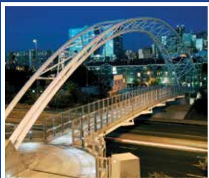
2007 NSBA Special Purpose Prize Bridge Award - 152 tons of 18" pipe curved in our Kansas City plant for the Highland Bridge. Denver, CO
