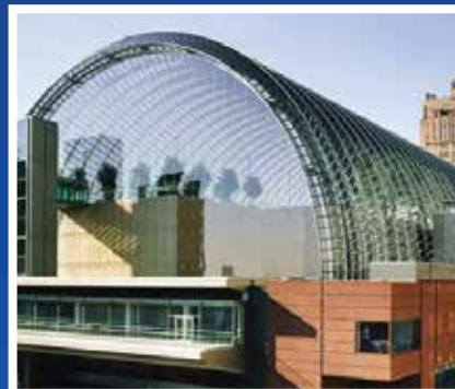
2003 IDEAS 2 National Winner - 300 tons of 5 inch square tubing curved 45° off-axis for the Kimmel Center. Philadelphia, PA
