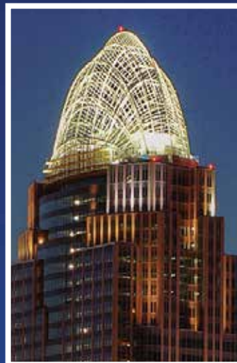
2012 IDEAS 2 Merit Award - 133 tons of 16 inch pipe curved for the Rooftop Tiara of the Great American Tower at Queen City Square. Cincinnati, OH
