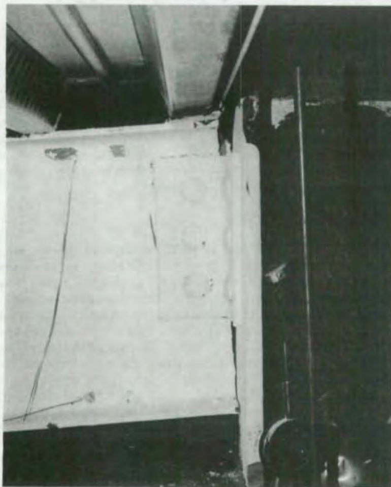
Figure 6 - End supports for test specimens.
