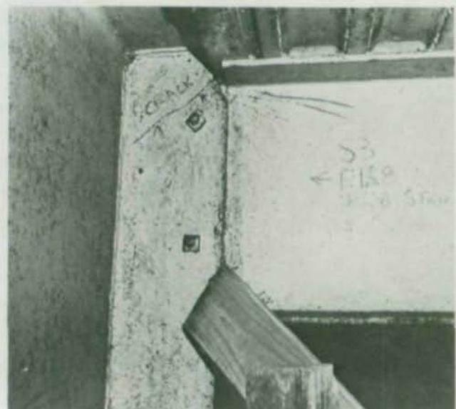
Fig. 36. Cracked rivet heads from cyclic end rotation
