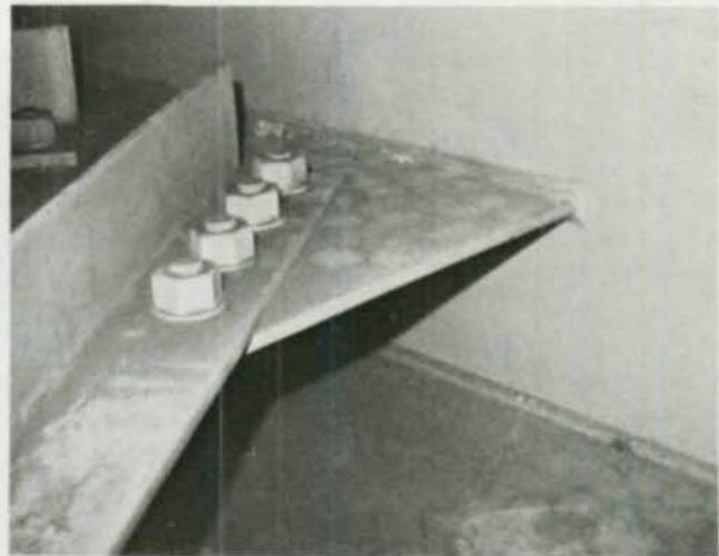
Fig. 59. Typical lateral bracing gusset without transverse stiffener plate
