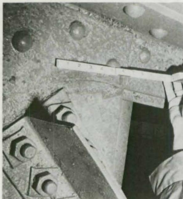
Fig. 61. Cracked riveted-bolted gusset caused by lateral bracing vibration
