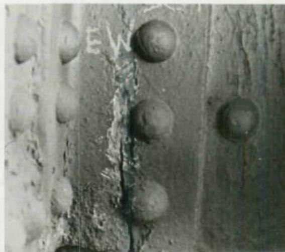
Fig. 35. Fatigue crack in standard connection angle
