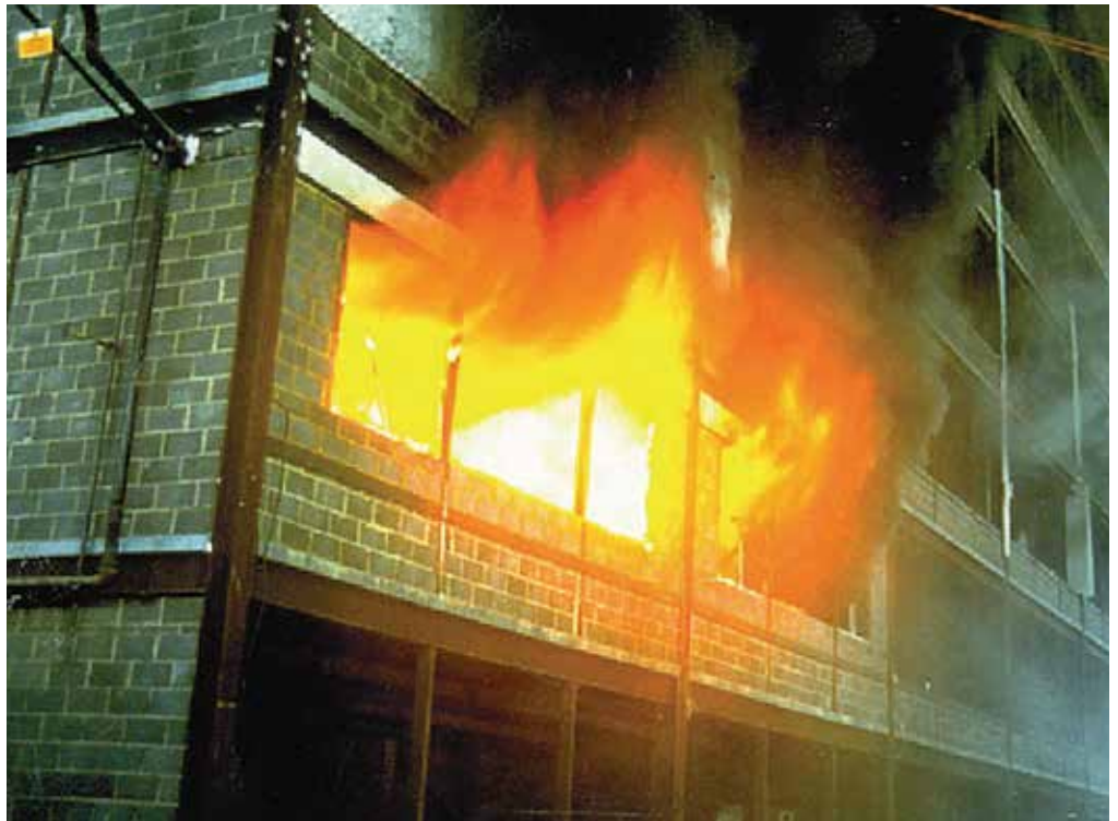
View of Cardington Test Building during fire exposure.
