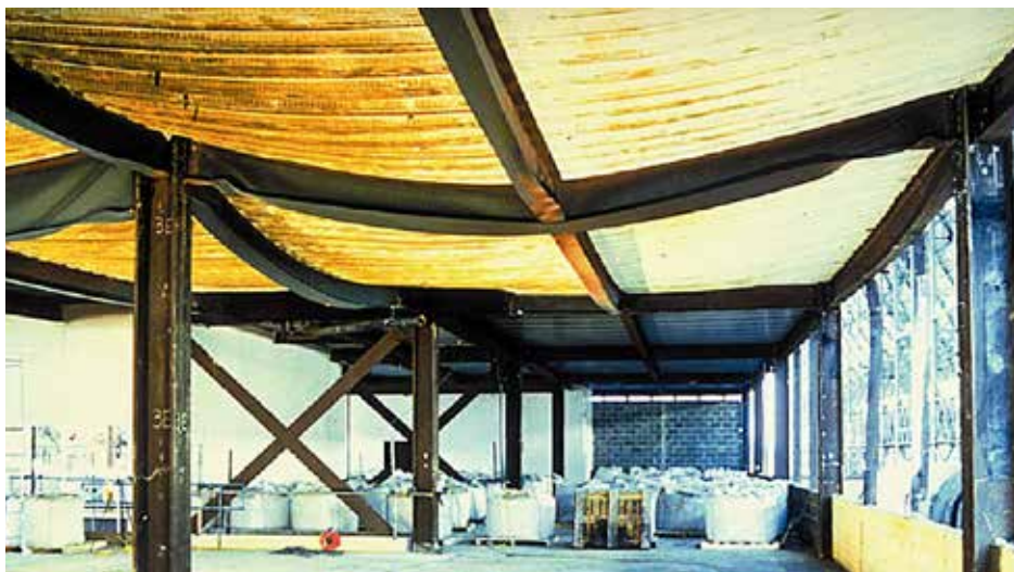
Beam in Cardington Tests after reaching temperature in excess of 1,600°F.
