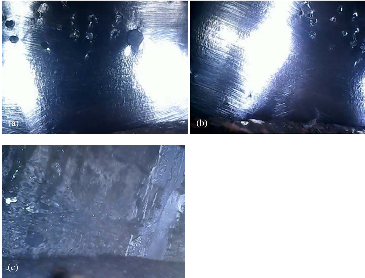
Figure A.90 – (a) First visible defects can be seen around the voids in specimen W24-BSW-T59-R100 during cycle 1, (b) the first folded steel defect can be seen at the bottom of the area with the glare during cycle 2, and (c) full fracture through the bottom of the specimen occurred during cycle 3 when the bottom of the specimen was in tension.
