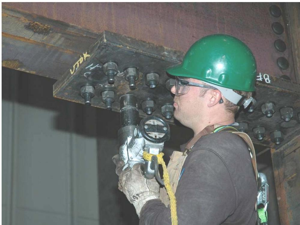
Figure 2.11 Bolt Tensioning
