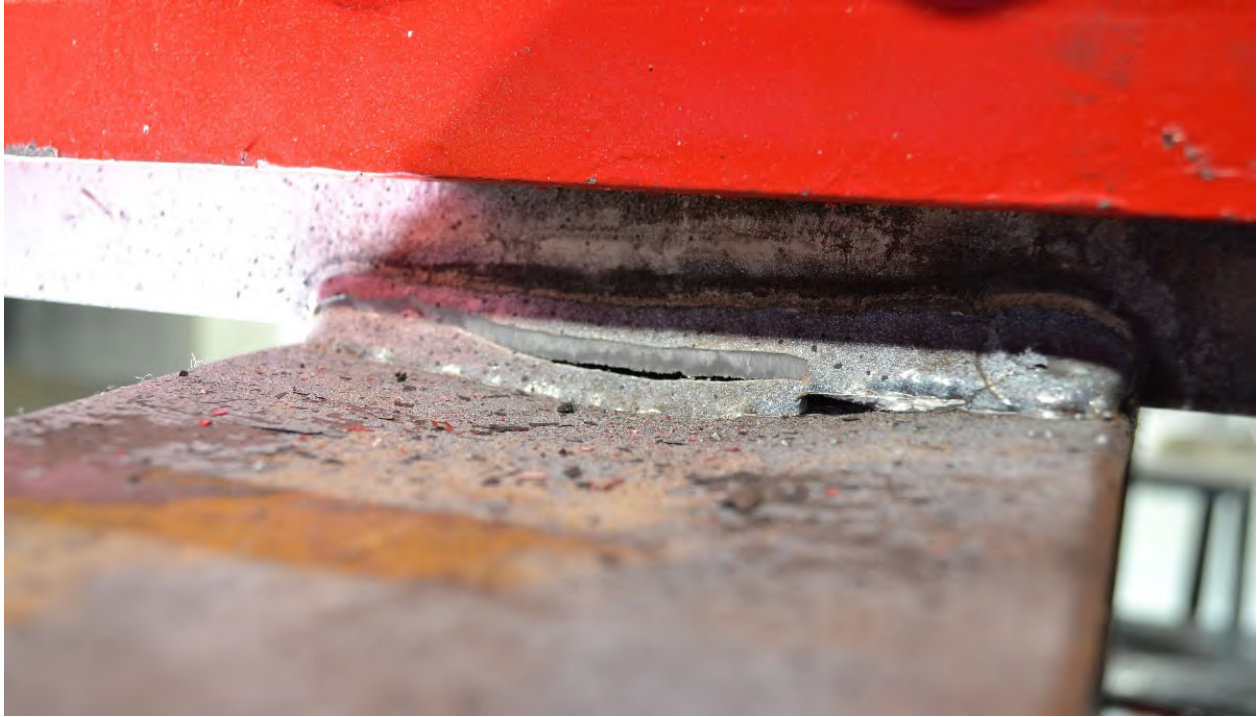
Figure A-137: Weld fracture of W16X31-ST-E3 after testing (Side 2)
