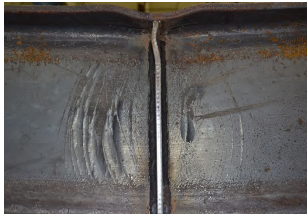
Figure 3.7-10: Comparison of web condition with eccentric and concentric stiffeners
