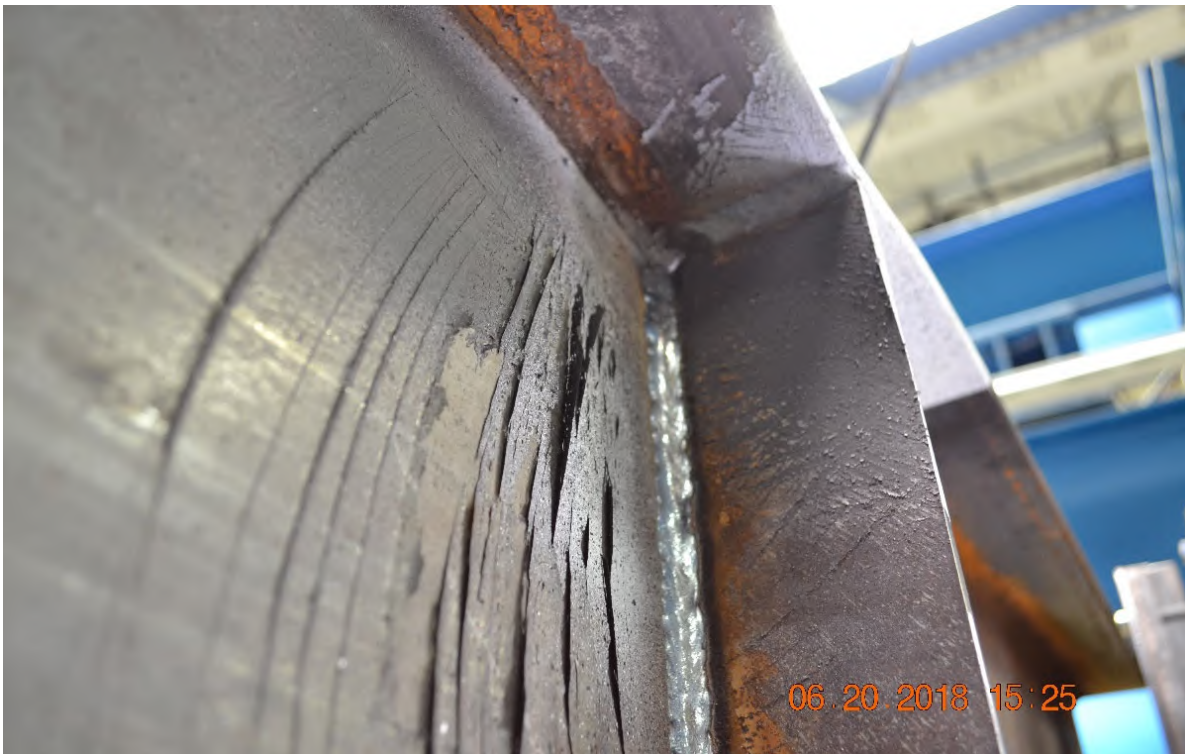
Figure A-69: Side view of W12X26-SC-E0 after testing emphasizing yielding
