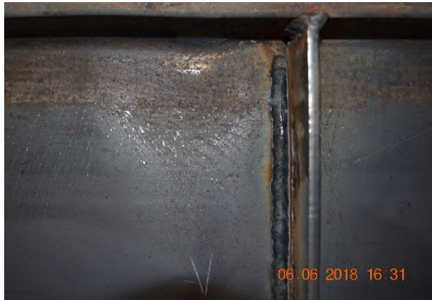
Figure 3.7-10: Comparison of web condition with eccentric and concentric stiffeners
