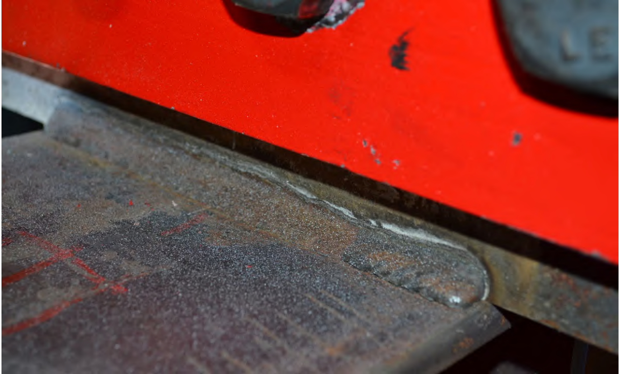
Figure A-154: Weld condition of W10X39-ST-E2 after testing (Side 1)
