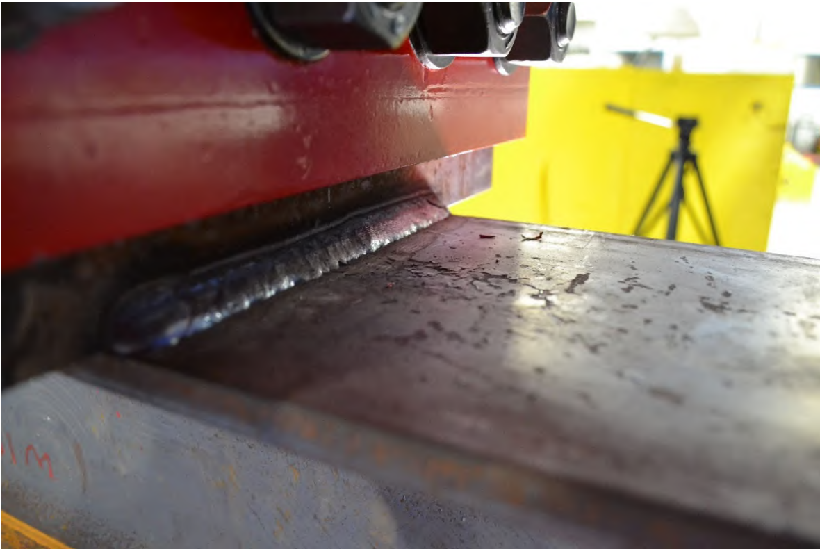
Figure A-145: Weld condition of W10X39-ST-NA after testing (Side 1)
