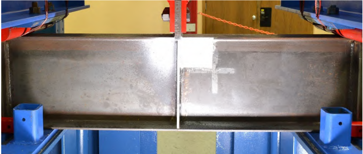
Figure A-139: Elevation of W16X31-ST-E0 after testing
