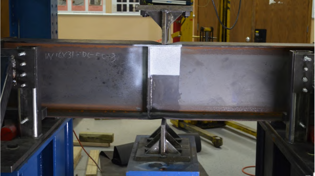
Figure A-80: Elevation of W16X31-DC-E3 after testing
