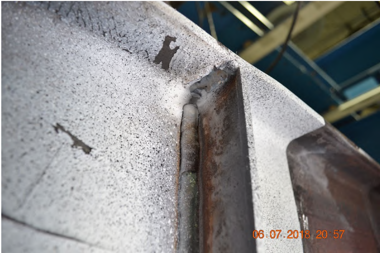
Figure A-35: W10X19-SC-E0 after testing emphasizing flange and weld yielding
