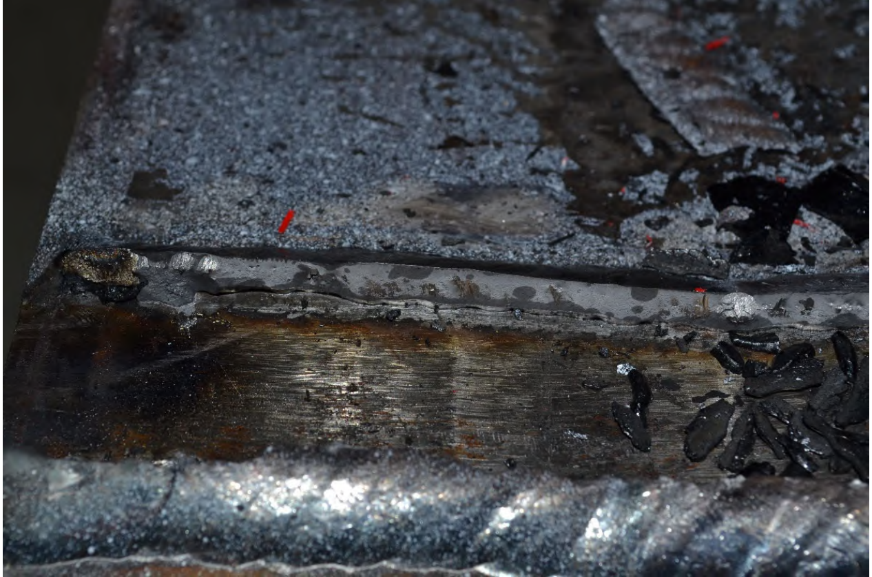
Figure A-167: Weld fracture of W12X26-ST-E4 after testing
