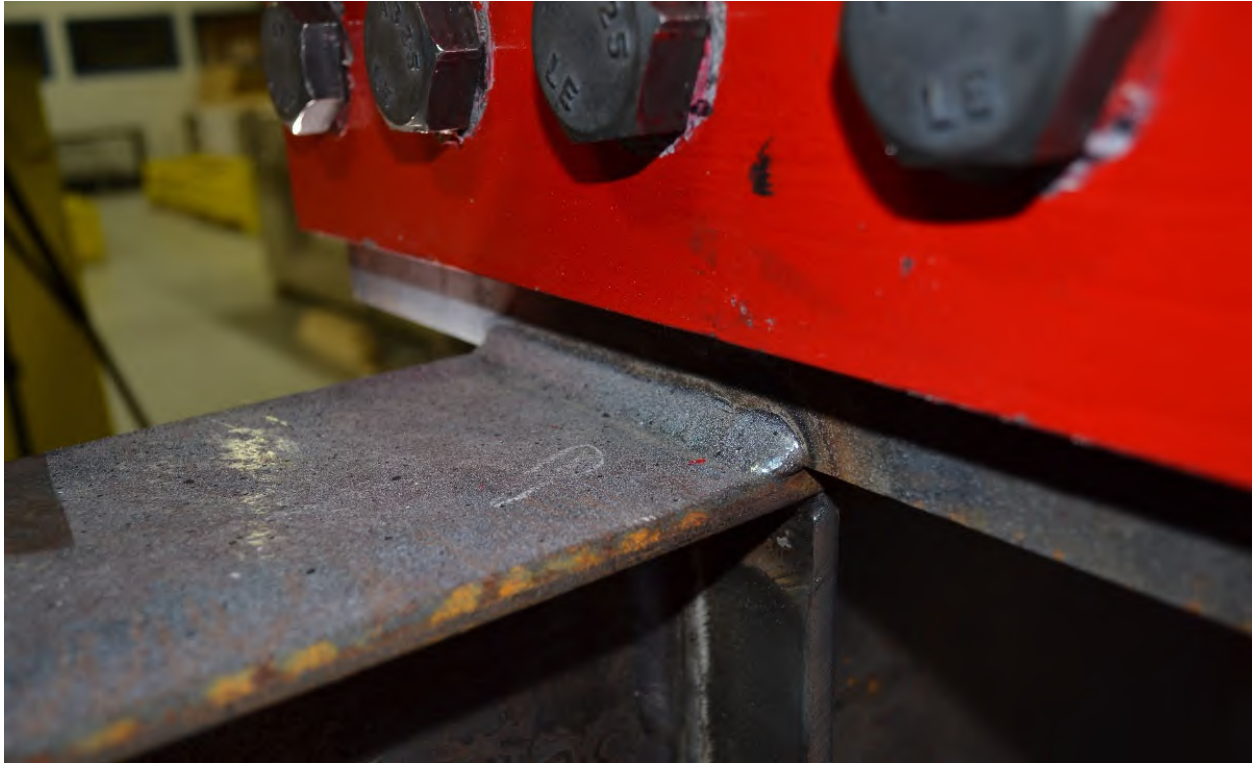
Figure A-140: Weld condition of W16X31-ST-E0 after testing (Side 1)
