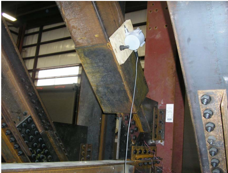
Figure 4 - Fully Bolted Buckling Restrained Brace Connection (prior to test)
