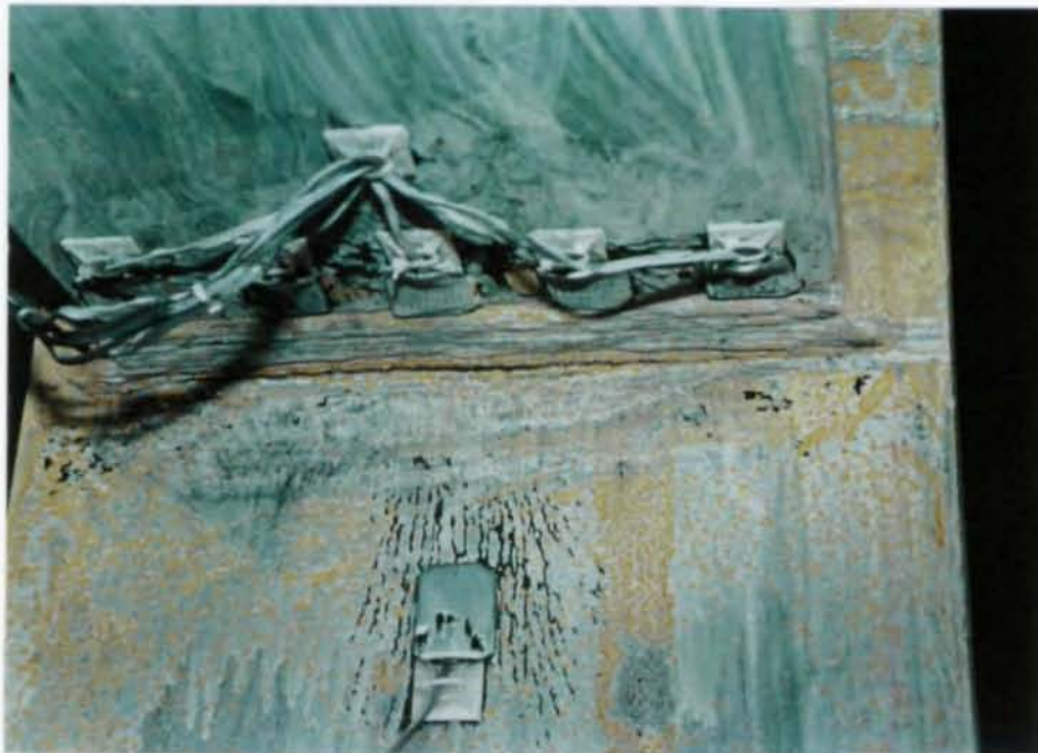
(b) Crack Initiation at Toe of Bottom Flange Groove Weld
