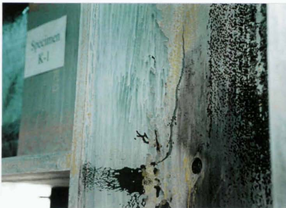
(b) Propagation of Column Fracture near k Area
