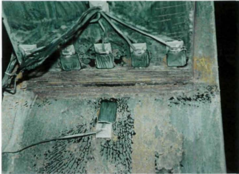
Figure 3.26 Specimen K3: Column Flange Fracture at Beam Bottom Flange Level (5% Drift, 1 st Cycle)
