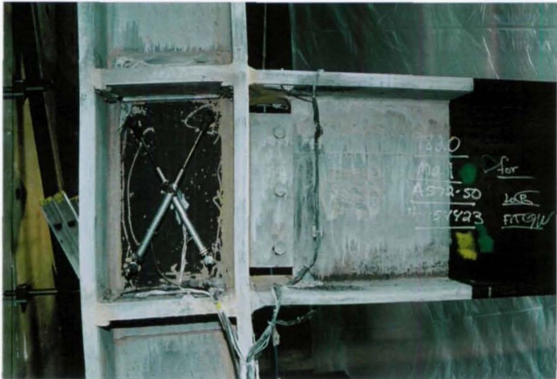
Figure 4.12 Specimen K5: Panel Zone Yielding at 5% Drift
