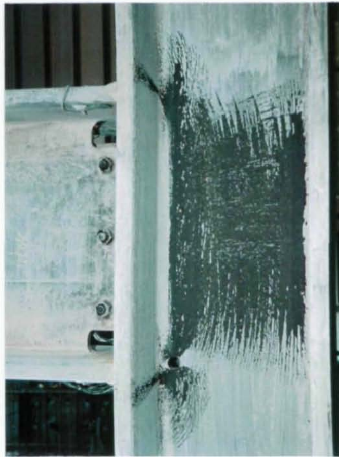
Figure 3.25 Specimen K3: Panel Zone Yielding Pattern at 3% Drift
