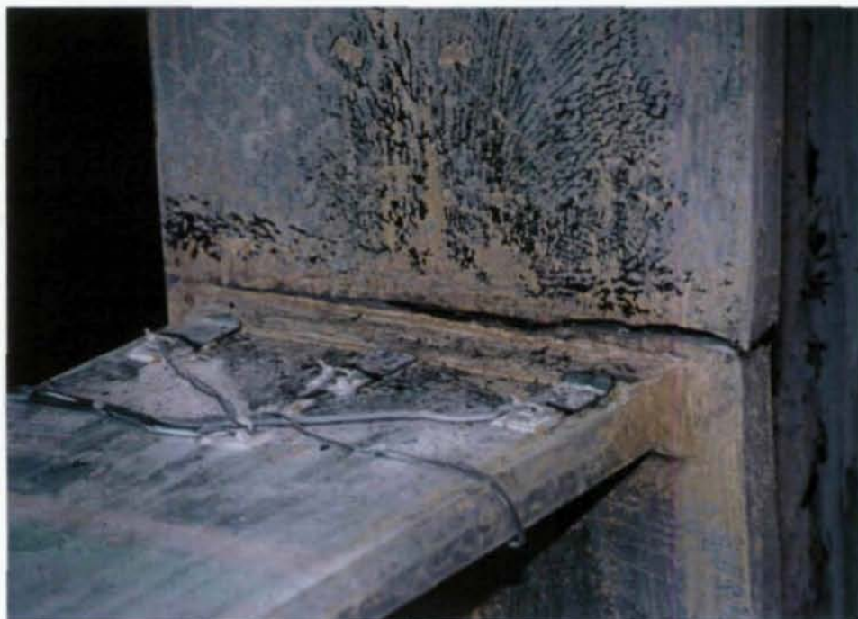
(a) Fracture of Column Flange
