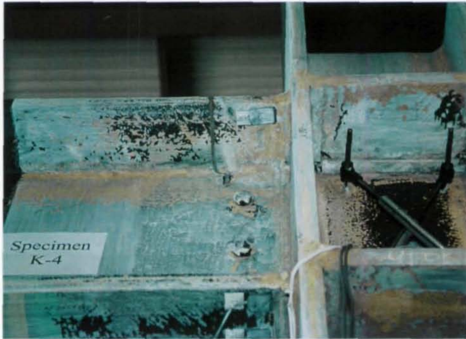
(a) Brittle Fracture of Beam Top Flange
