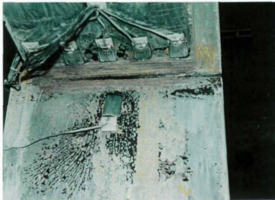
Figure 3.27 Specimen K3: Column Flange Fracture at Beam Bottom Flange Level (5% Drift, 2 nd Cycle at 3.14 in)
