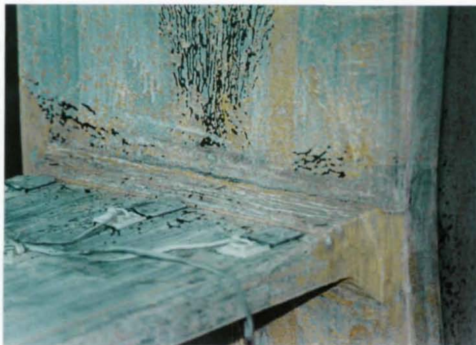
Figure 3.4 Specimen K1: Crack at Toe of Top Flange Groove Weld (10 in. Beam Deflection)
