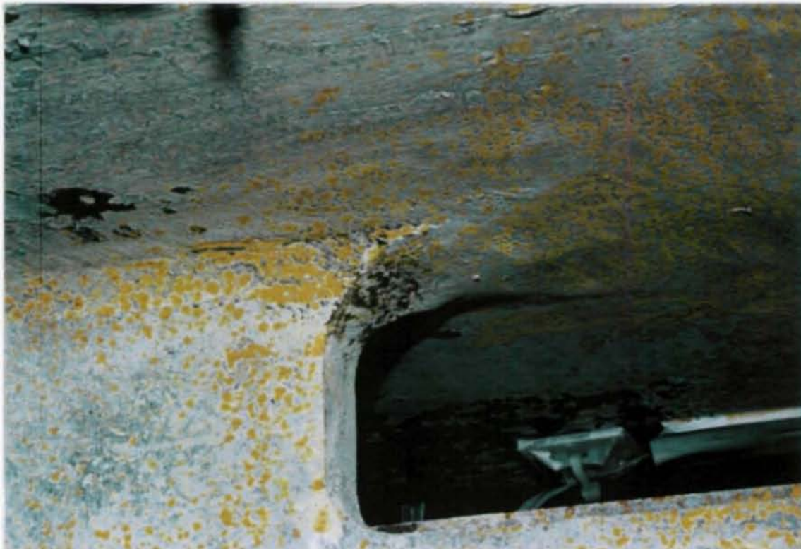
Figure 4.13 Specimen K5: Crack Initiation in Top Flange Weld Access Hole at 5% Drift
