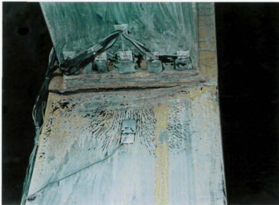
(a) Fracture of Column Flange
