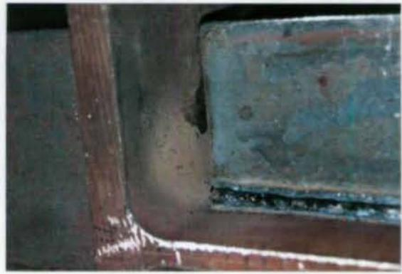
**Figure 5d** Type III Web Gap Detail.
