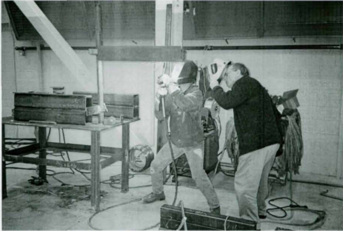
Figure 20. Overhead Welding of Test Specimen at Walters Inc.
