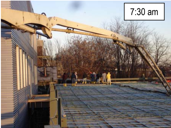
Figure 5.2 Placing concrete: November 22, 2006.
