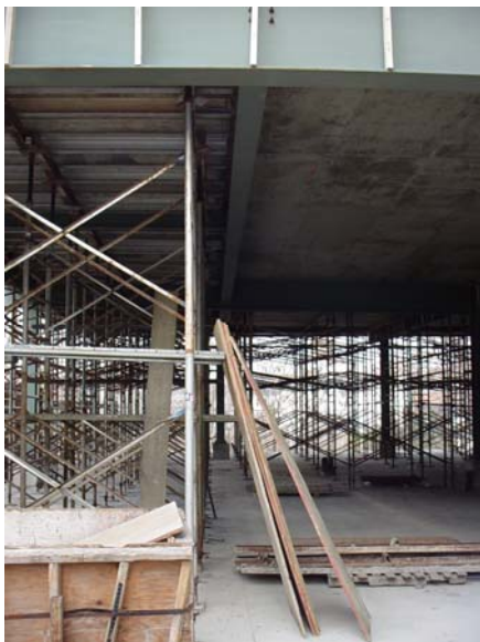
Figure 5.4 Shoring condition at Beam B: December 14 through 19, 2006.
