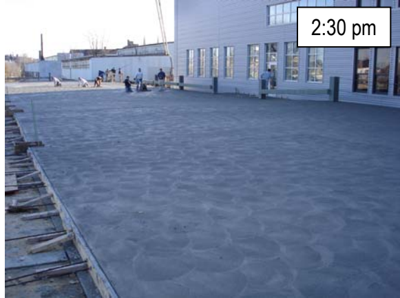
Figure 5.2 Placing concrete: November 22, 2006.
