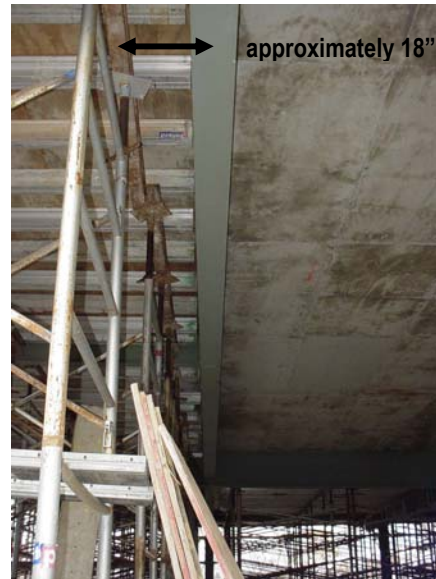
Figure 7.1 Location of form shores at Beam B (photo taken as shores are being removed and coincides with the photo shown in Figure 5.4).
