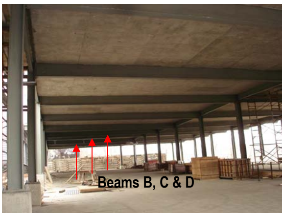
Interior of parking structure.
