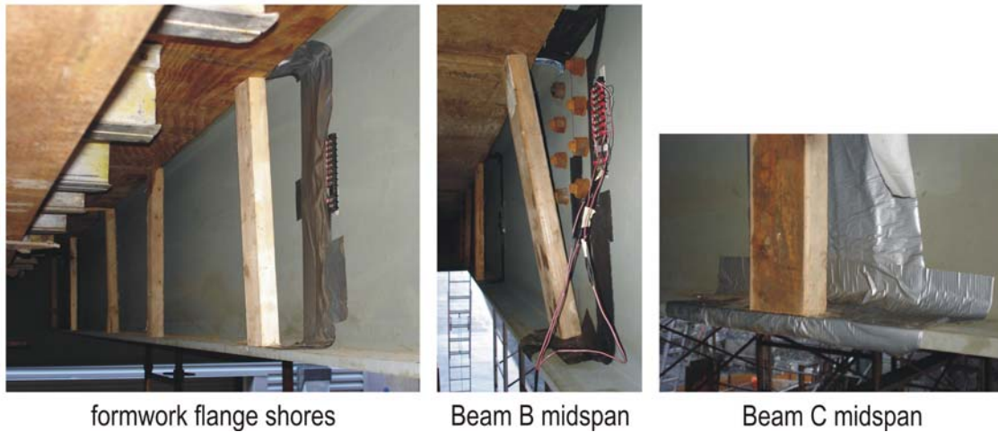
Figure 4.3 Installations of formwork shores near and directly on top of strain gages.
