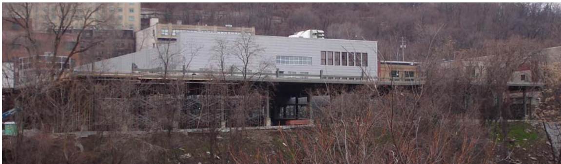
Overall view of 11 bay parking structure looking West from across railway right-of-way.
