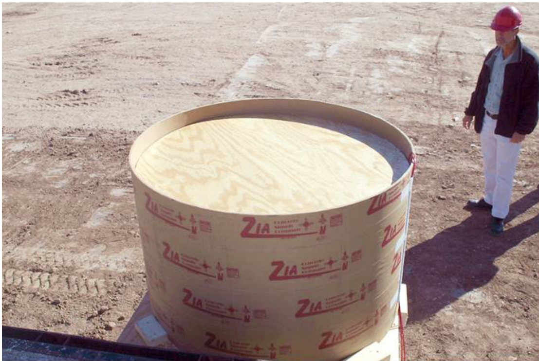
(b) ANFO is then completely filled and capped with plywood.
