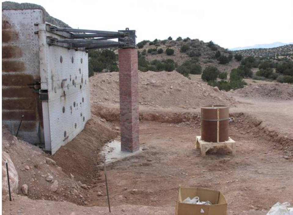
(a) South view of the test article.
