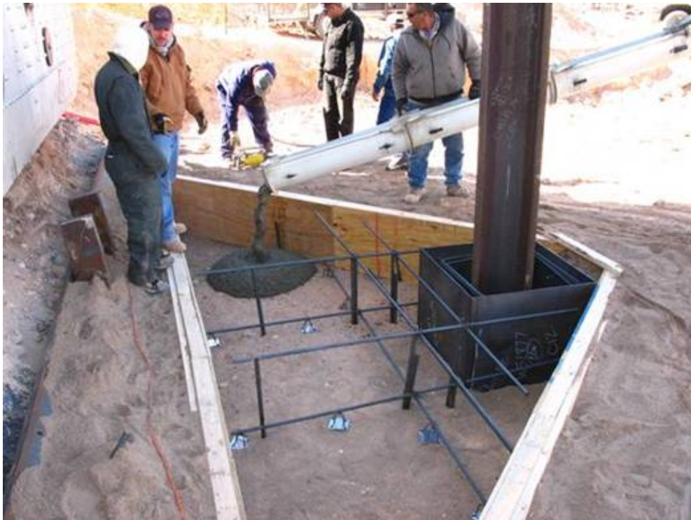
(b) Pouring of the base concrete.
