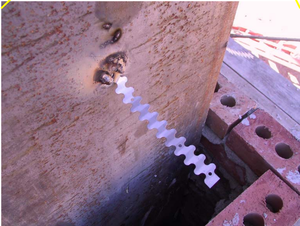
(b) Close-up view of wall tie attachment to column.
