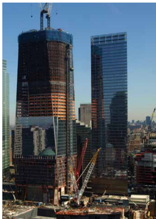
Figure 1 150 North Riverside, New York, NY structure uses high strength structural steel (HS3) of 70 ksi (485 MPa), completed in 2017 (Finnigan et al. 2015)
