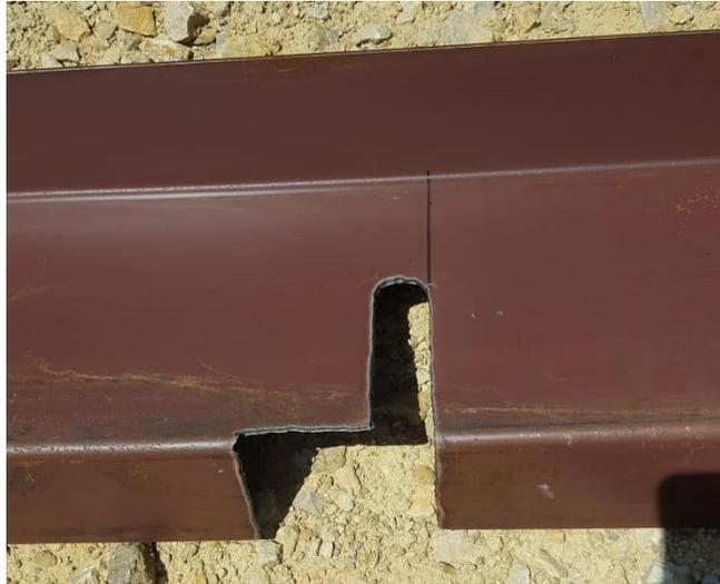
Fig. 7- 2: Purlin flange and web profile cut-out
