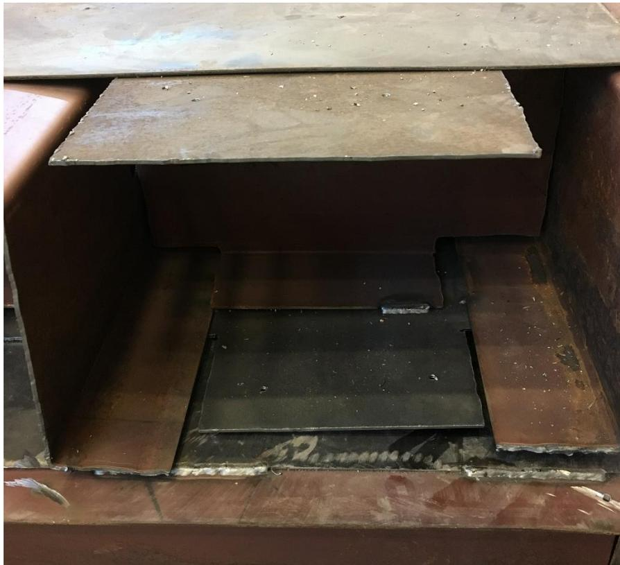
Fig. M -10. Center panel with top and bottom plate notches for joining with edge panels
