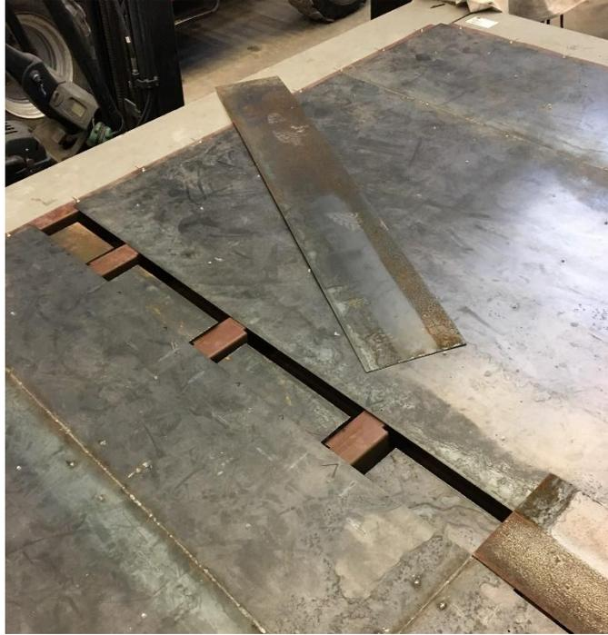
Fig. 7- 7: Splice plates being installed over the splice seats of the center-top plate and the top plate of the exterior panel
