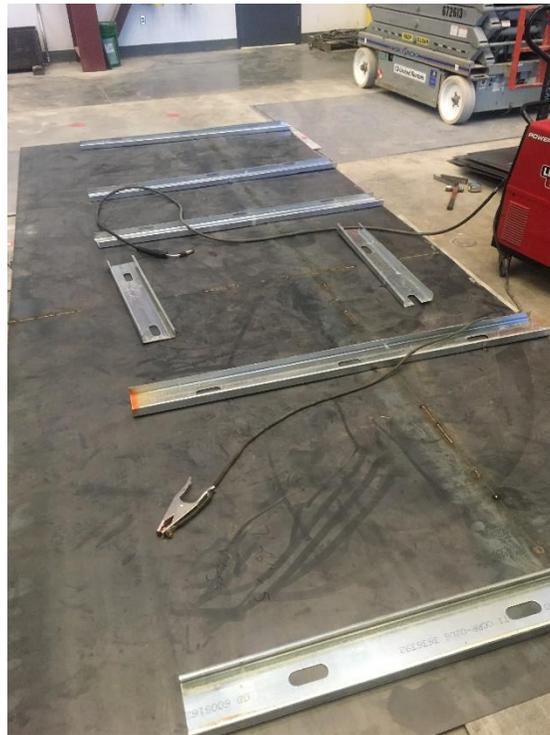
Fig. M -6. Typical process of welding top and bottom plates with stiffeners to reduce warping
