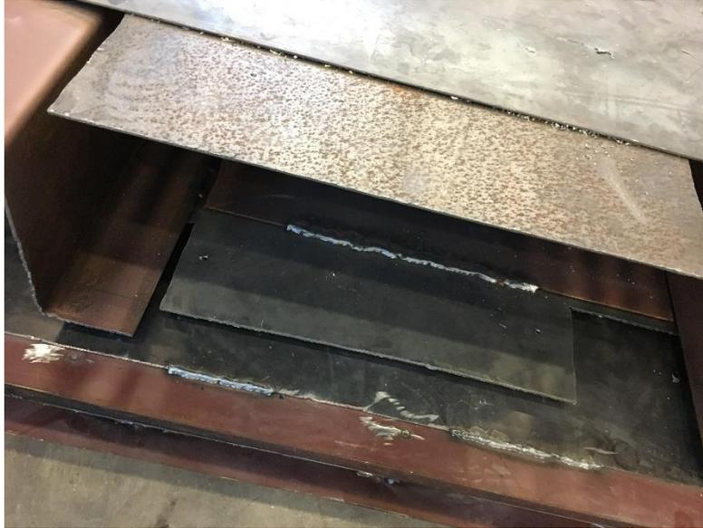
Fig. 7- 4: Notched bottom plate of the center panel and top plate lap-splice pieces
