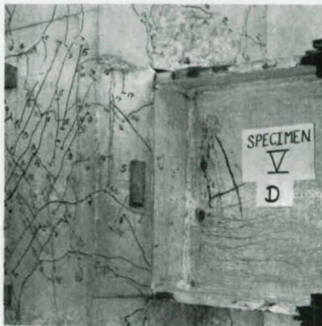
Fig. 4.18 Joint 5 after failure. (Top flange in compression in L1 and U1)
