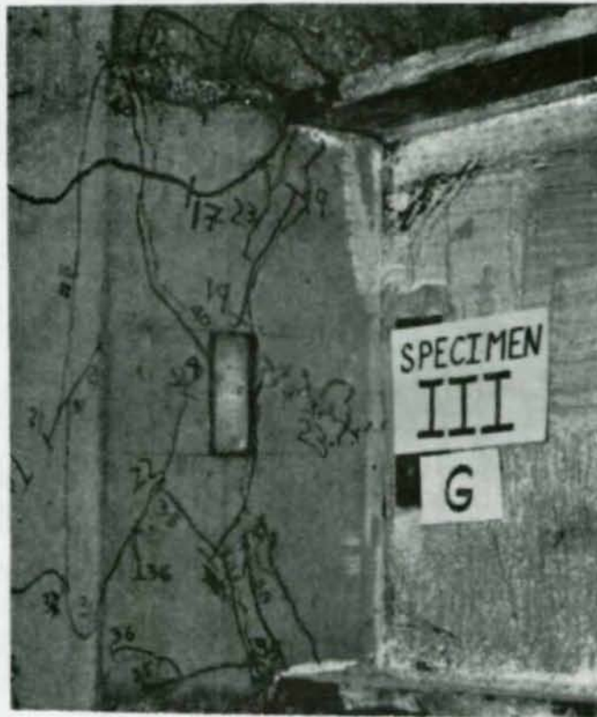
Fig. 4.10 A view of joint 3 after failure. (Top flange in tension in L1 and U1)
