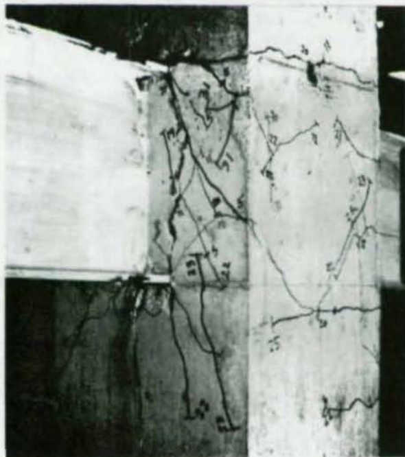
Fig. 4.5 A view of joint 1 after failure. (Upper left flange in tension in cycles L1 and U1)
