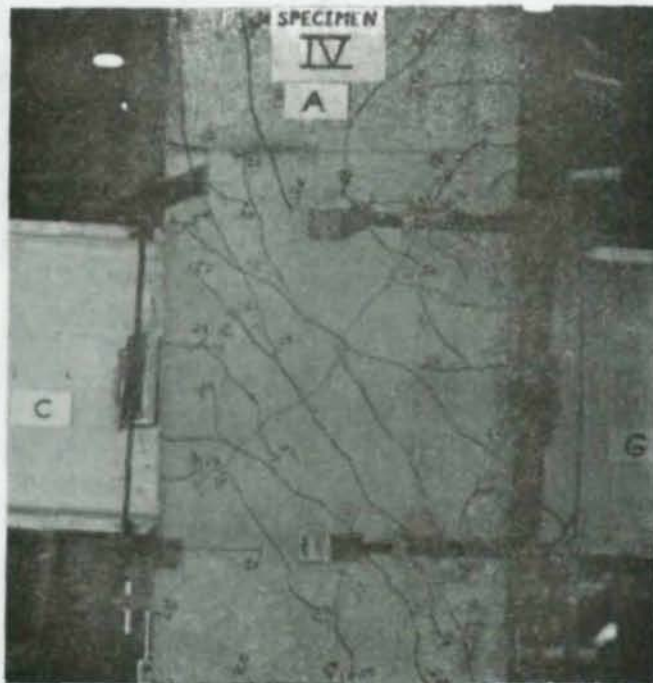
Fig. 4.13 Joint 4 after cycle U1. (Upper left flange in compression)
