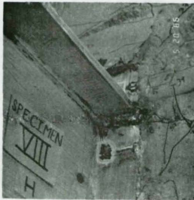
Fig. 4.32 Joint 8 after failure. (Top flange in compression in L1 and U1)
