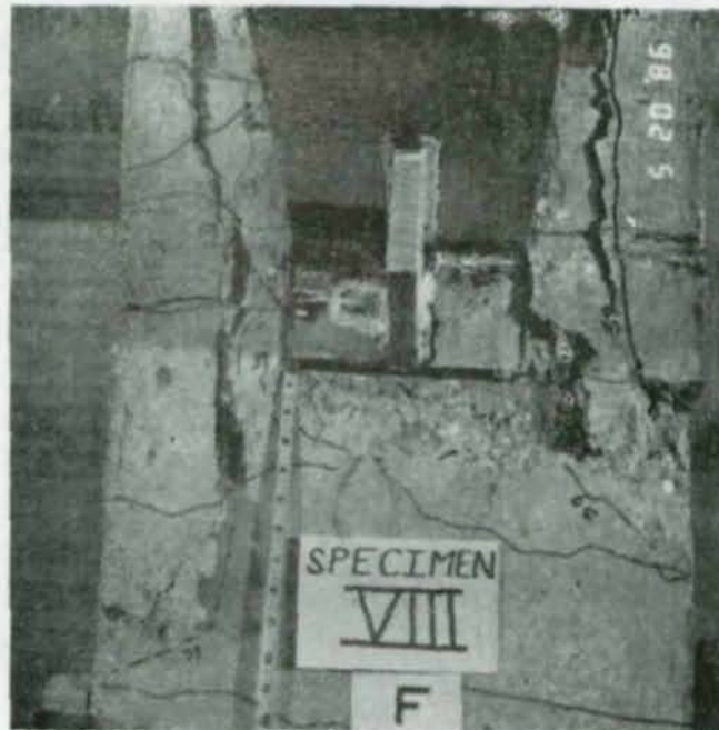
Fig. 4.31 Joint 8 after failure. (Bottom flange in compression in L1 and U1)
