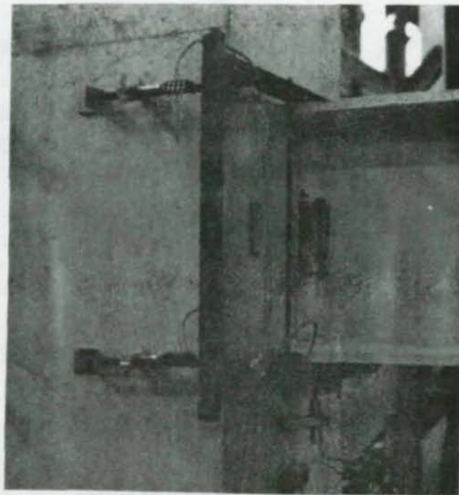
Fig. 3.26 Steel frame to measure joint distortion.
