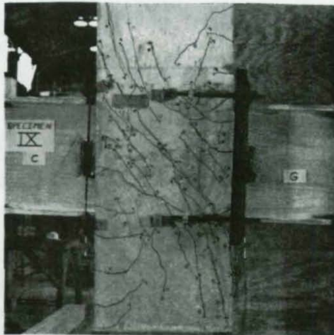
Fig. 4.34 Joint 9 after cycle U1. (Upper left flange in compression)
