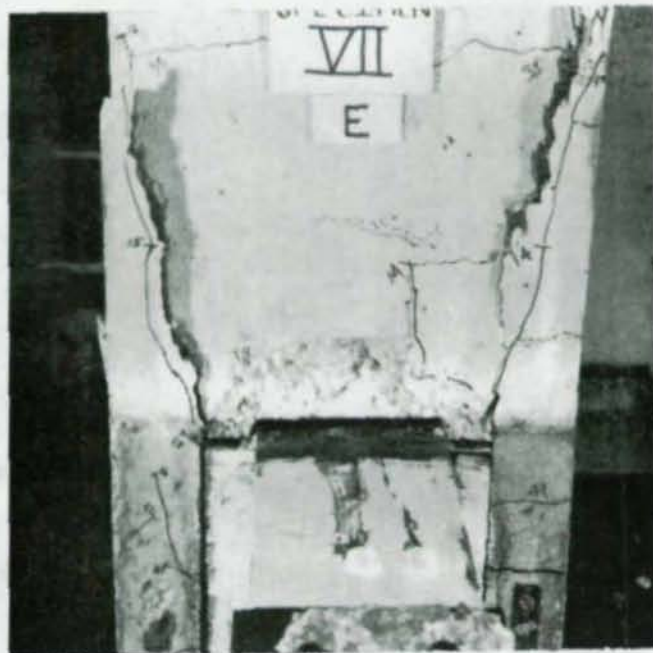
Fig 4.26 Joint 7 after failure. (Top flange in compression in L1 and U1)
