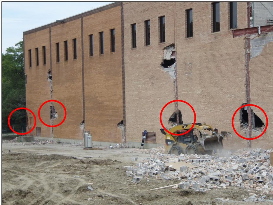
Figure 2.5- The Circled Columns on North Side of the Building were Removed During the Experiment.
