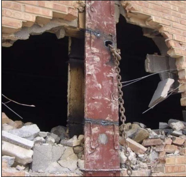
Figure 3.6- Torched Column Ready to be Pulled Out.
