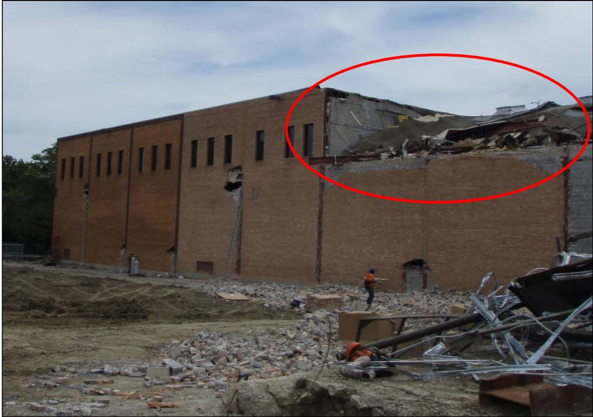
Figure 2.6- The Rubble Mass is Circled on the North Side of the Bankers Life and Casualty Company Building.
