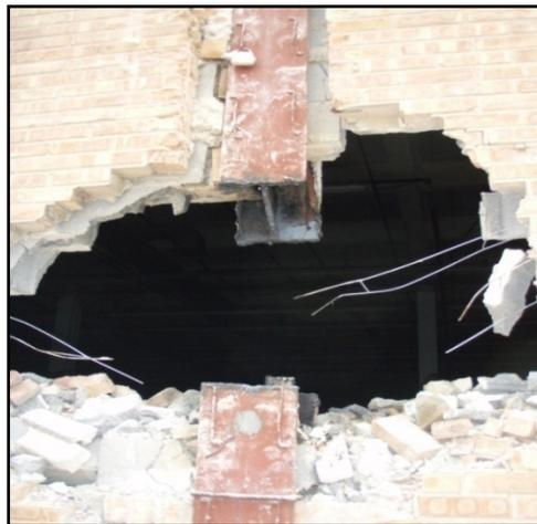
Figure 3.9- Column 16C Removed.
