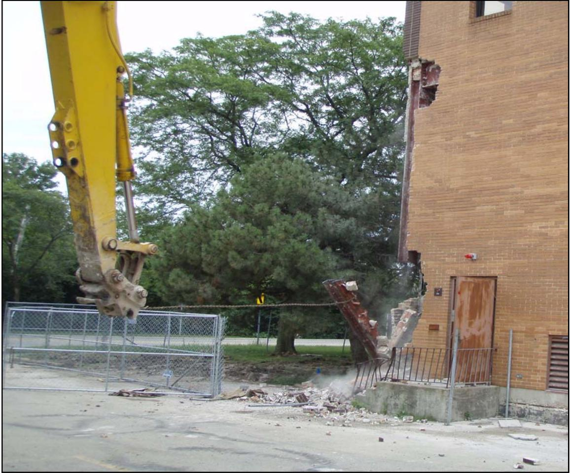
Figure 3.10- Torched Section of Column 11C Being Removed.
