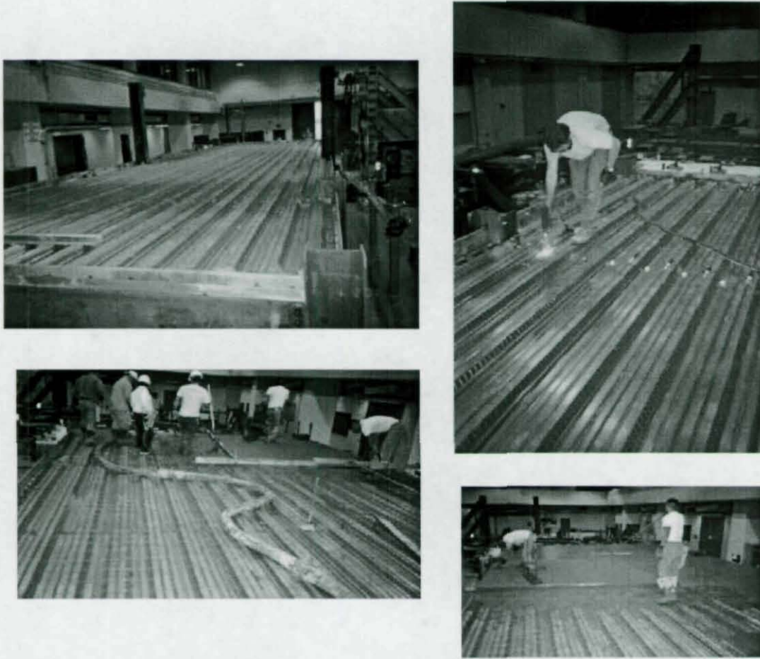
Figure 2.10. Construction of Test Structure
