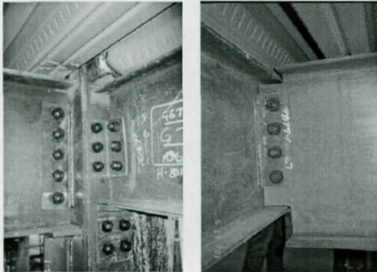
Figure 2.8. Beam-to-Column and Beam-to-Beam Connections
