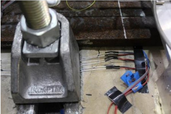
Concrete crack adjacent to Clamp 2
