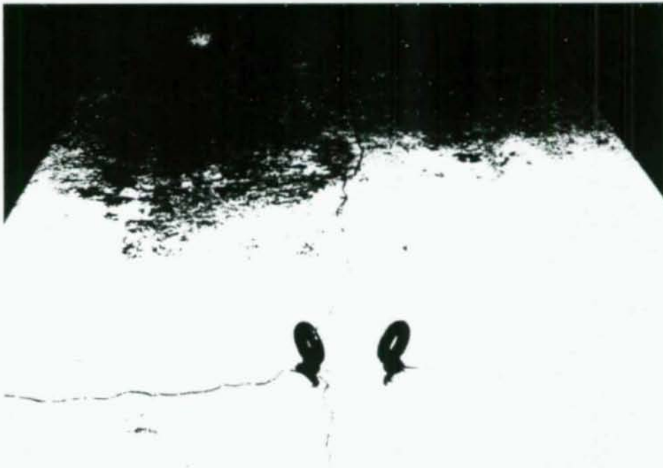
Figure 12: Cracking in concrete slab after the test
