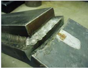
Welded cover plate detail
