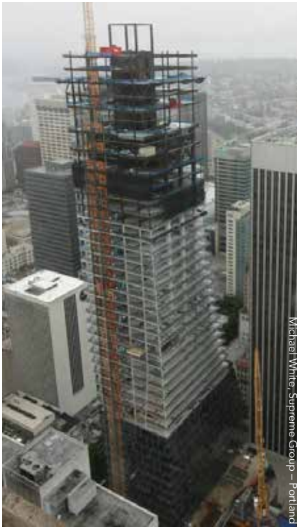
Rainier Square Tower in downtown Seattle, the first building to use the SpeedCore system.
