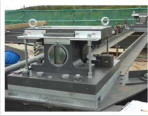
Bearing installation
