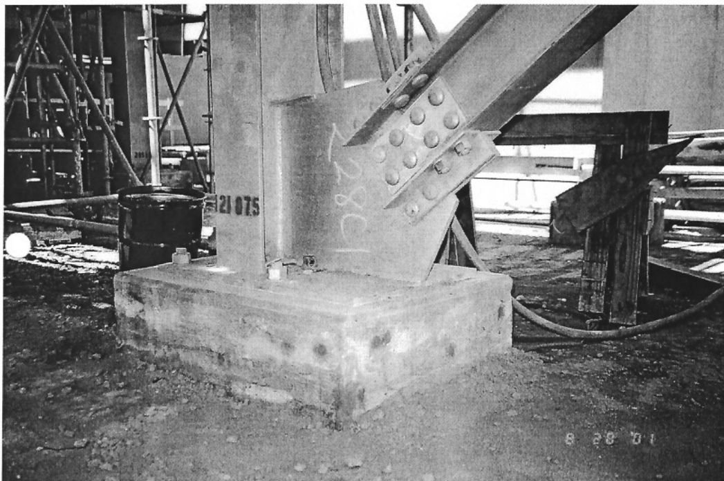
Fig. 2.5. Special detail for gusset plate and exposed base plate in a braced frame [courtesy of R. Drake, 2003]
