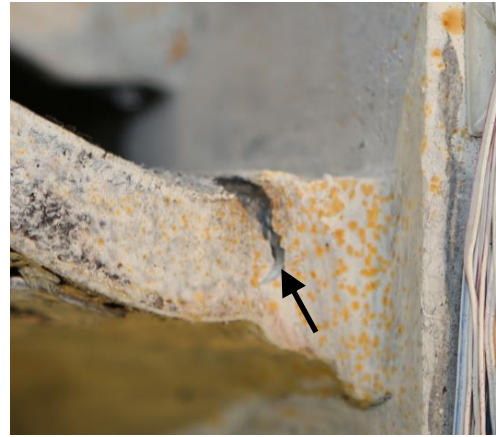
(b) Weld Fracture
