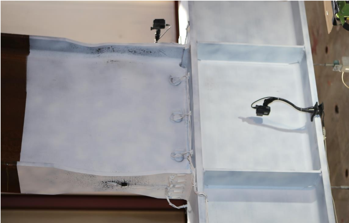
Figure 4.76 Specimen C6: Beam Web and Flange Local Buckling at +0.04 rad (2 nd Cycle)
