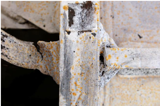
(c) East Beam Bottom Flange
