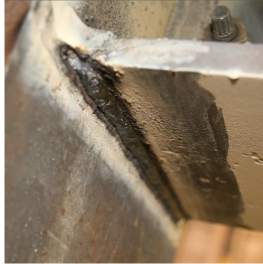
(b) Reinforcing Fillet
