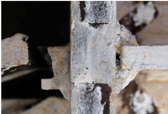
(a) East Beam Top Flange
