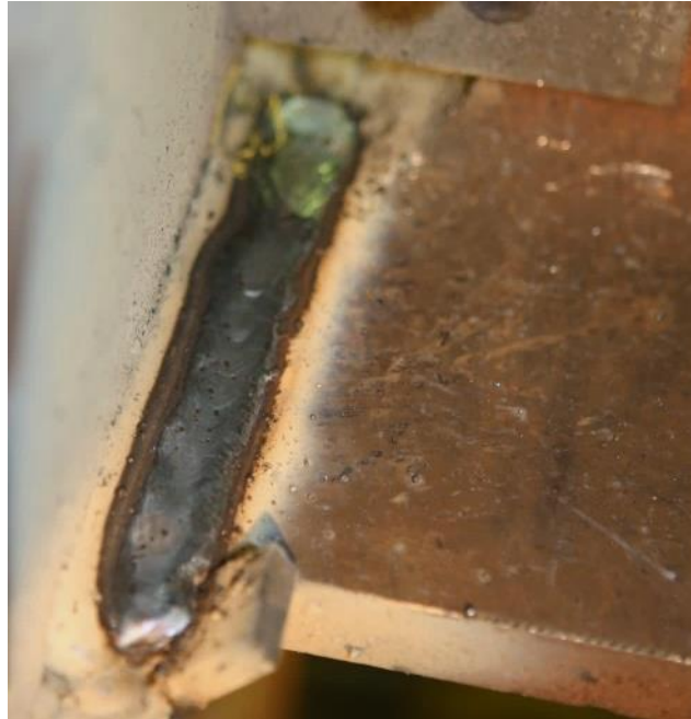
(a) Beam Bottom Flange
