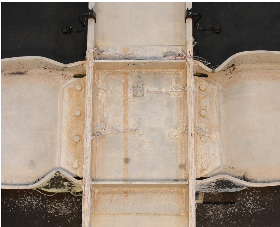
Figure 4.215 Specimen W3: Flange Local Buckling at -0.05 rad (1 st Cycle)
