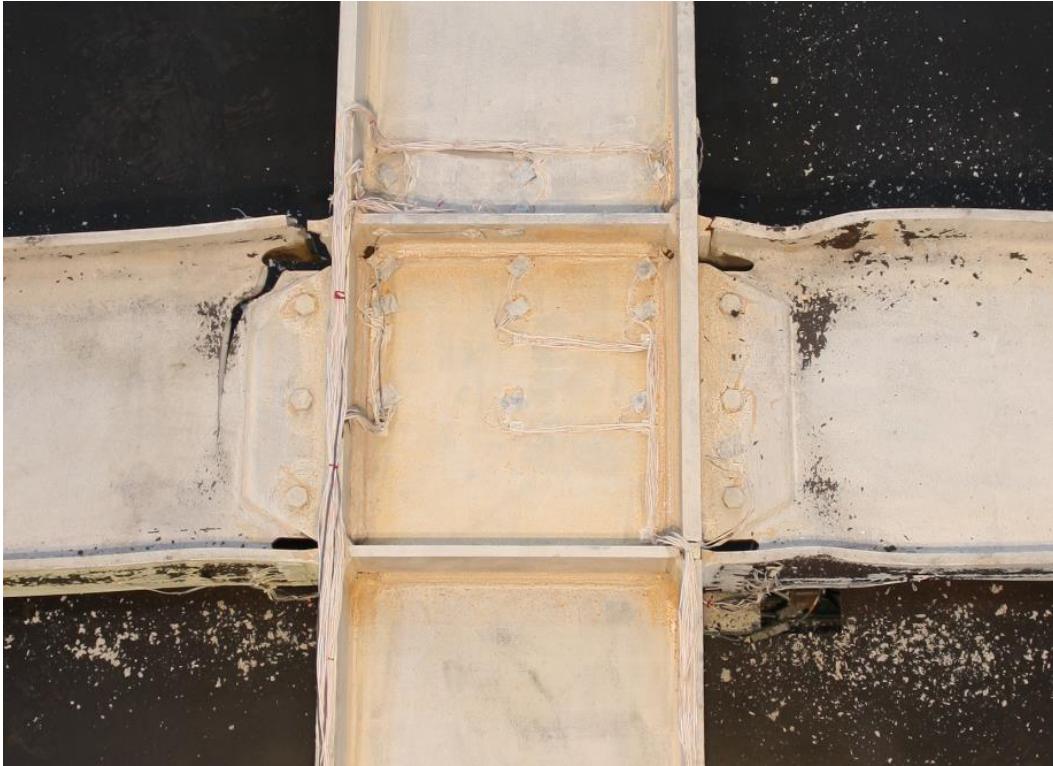
Figure 4.258 Specimen W4: Connection at End of Testing
