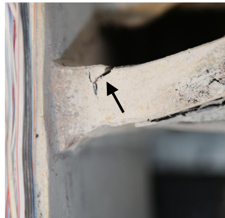
(b) Weld Fracture
