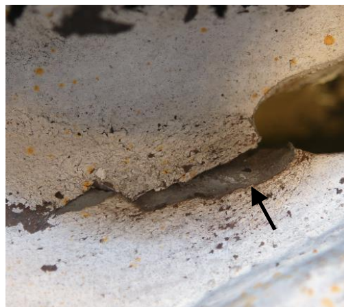
(b) Weld Fracture
