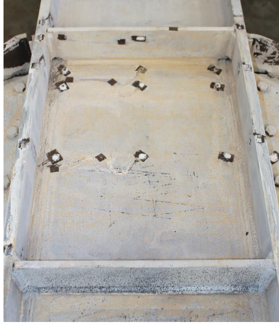
Figure 4.186 Specimen W2: Panel Zone (End of Test)
