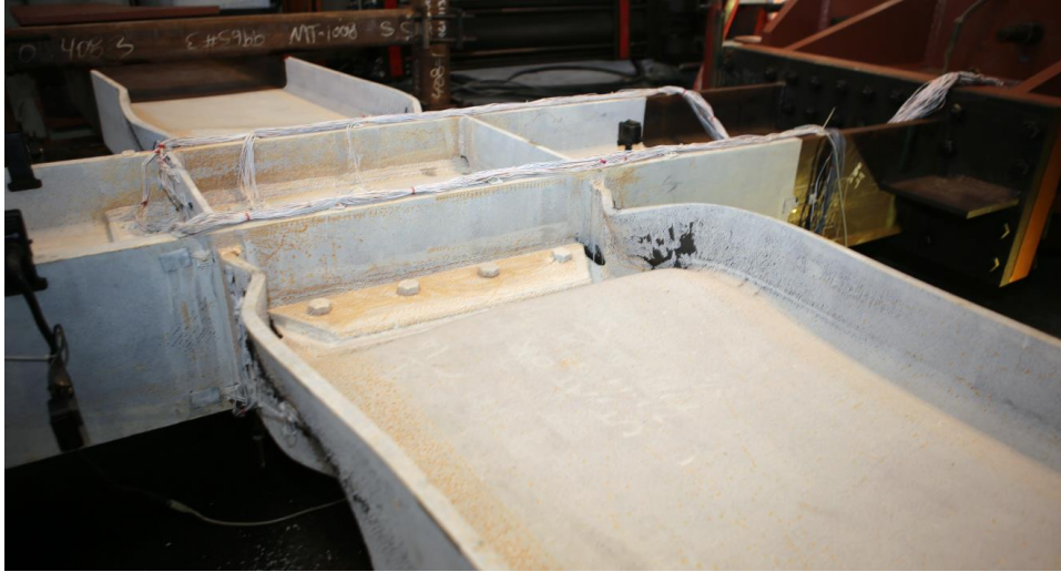
Figure 4.214 Specimen W3: Web Local Buckling at +0.05 rad (1 st Cycle)
