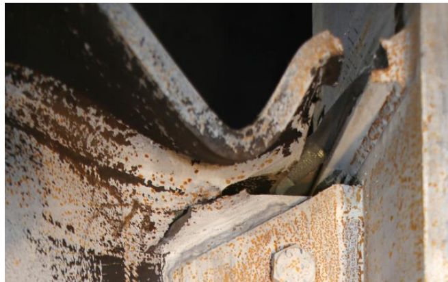
Figure 4.217 Specimen W3: East Beam Top Flange Weld Access Hole Tear
