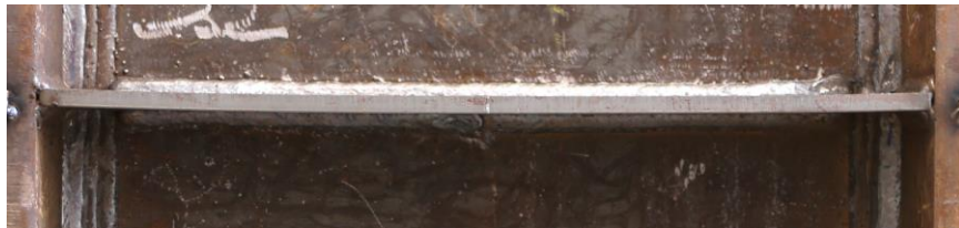
(b) Bottom Flange Continuity Plate
