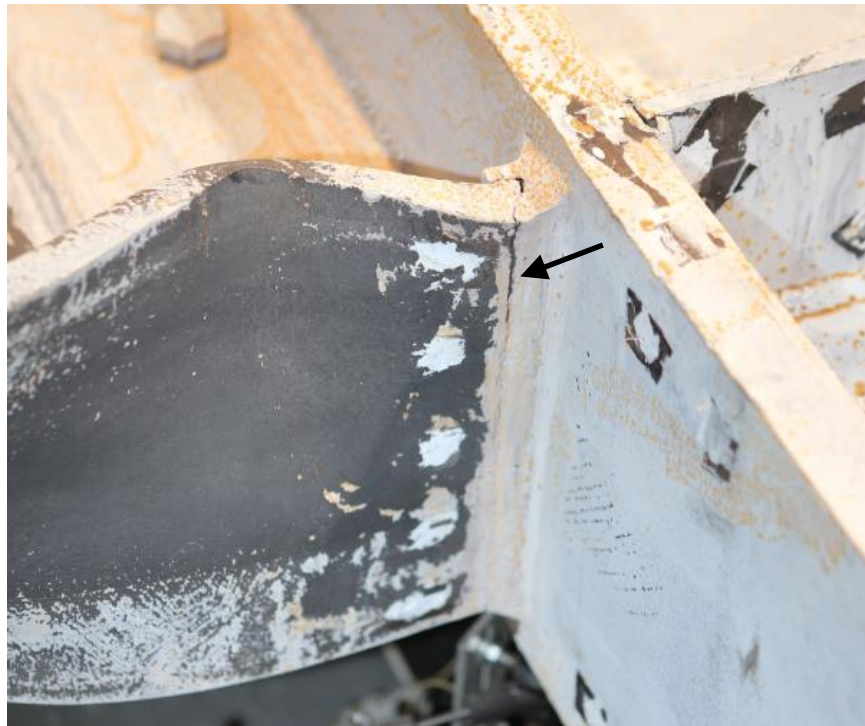
Figure 4.221 Specimen W3: West Beam Top Flange (End of Test)
