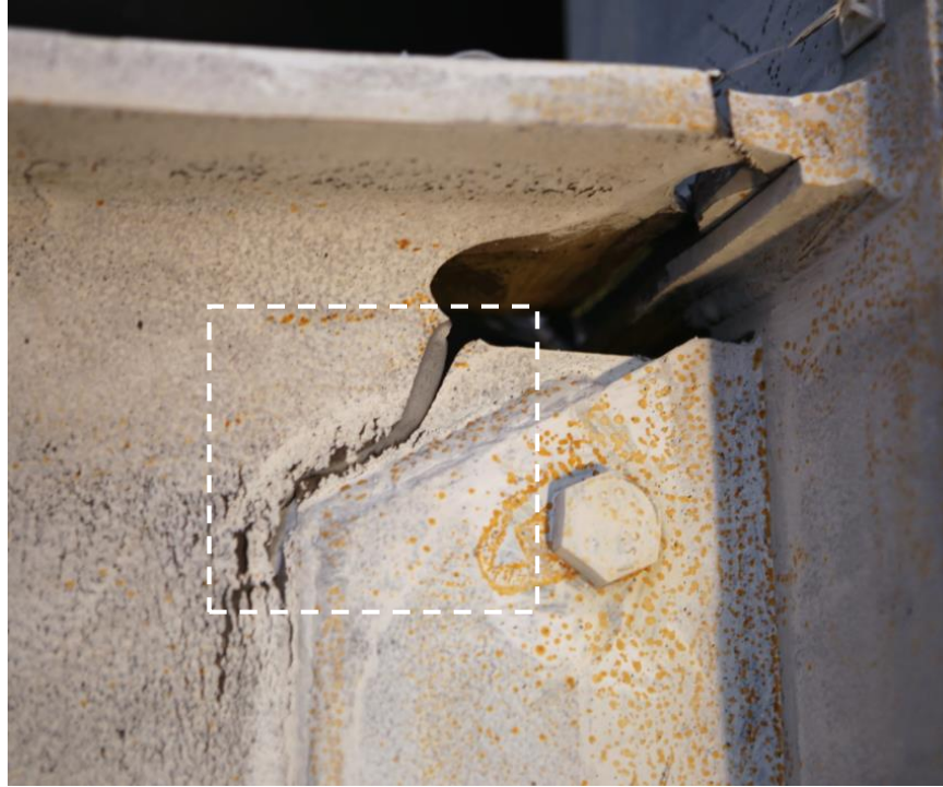
Figure 4.255 Specimen W4: East Beam Top Flange Weld Access Hole Fracture during First of -0.05 rad
