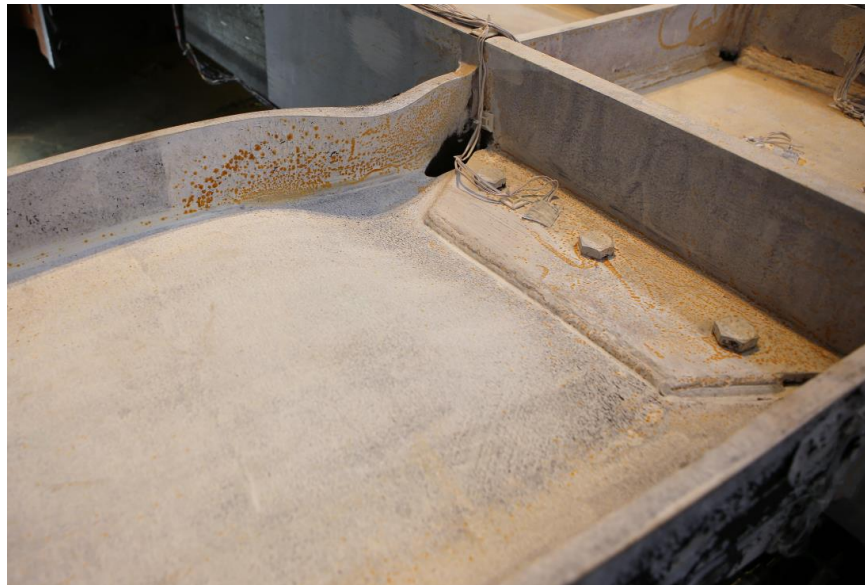
Figure 4.250 Specimen W4: West Beam Web Buckling at +0.04 rad (1 st Cycle)
