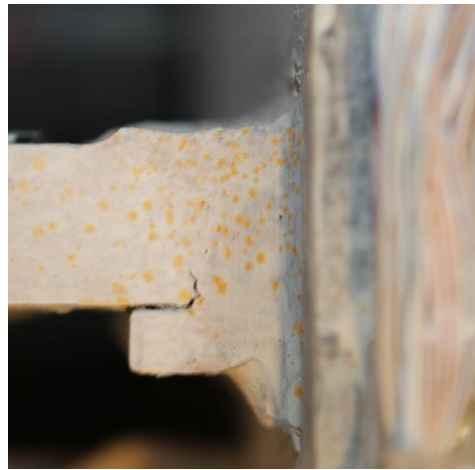
(b) Weld Fracture
