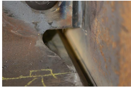
(b) Weld Access Hole
