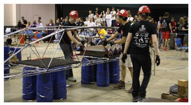
Stacked plastic buckets can be used as safety supports under decking.
