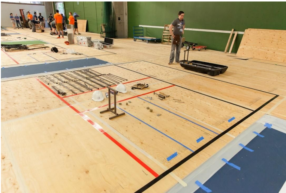
Staging area with bridge ready to go
